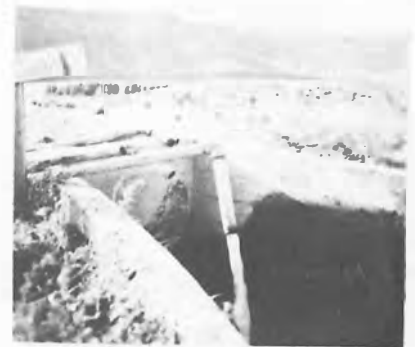
Vents at Inlet to Siphon
