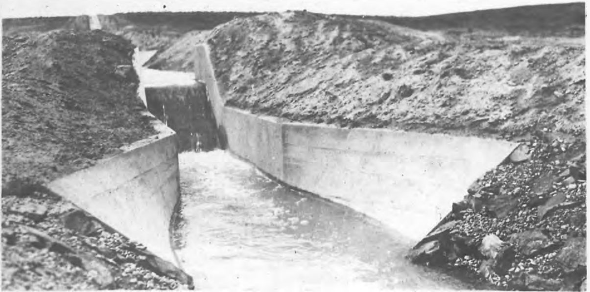
Figure 4 - Rectangular Inclined Drop at Oghee South Canal Lateral 5.7 - 2.5, Station 122+25
