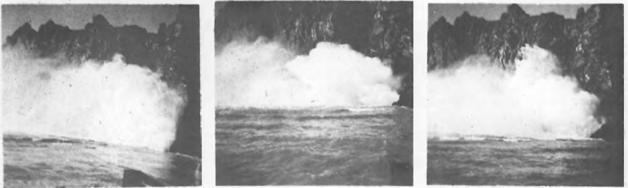
FIGURE 21 - DISTURBANCE DUE TO SURFACE WAVES IN STILLING POOL COLLIDING WITH HIGH-VELOCITY STREAM FROM OWYHEE SPILLWAY TUNNEL. DISCHARGE 3,000 SECOND-FEET
