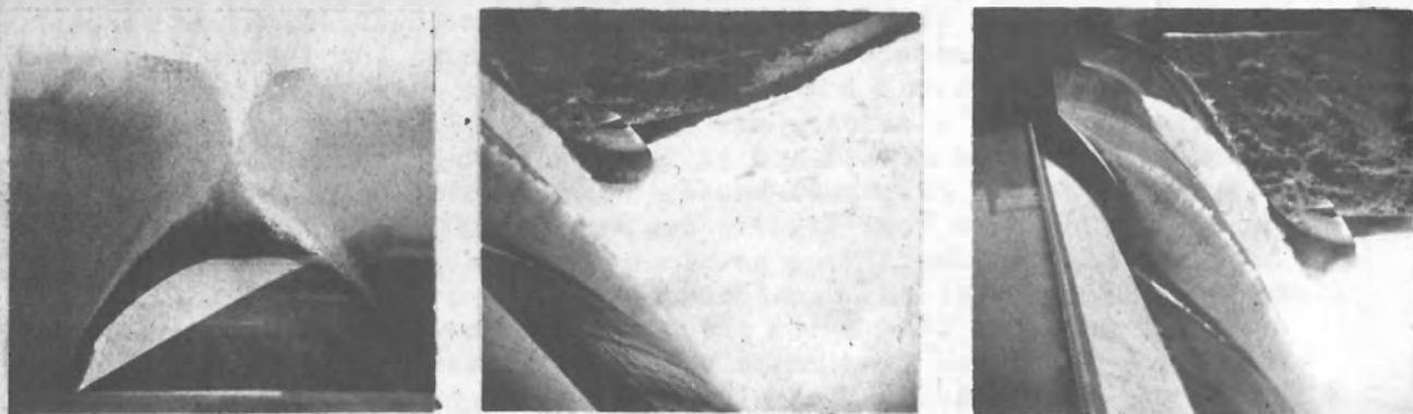
FIGURE 23 - TWO LEFT DRUM GATES AT BLACK CANYON DAM HALF LOWERED
