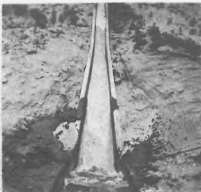
FIGURE 10 - CHUTE ON OWYHEE NORTH CANAL LATERAL 43.6
