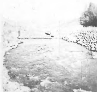
Rock Fill Opposite End of Lined Pool to Check Erosion
