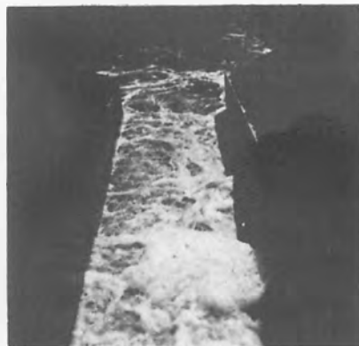
Figure 6 - Flow Conditions in Inclined Rectangular Drop at Station 313+55 on Owyhee South Canal Lateral 5.7 - 2.5
