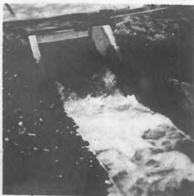
Figure 6 - Flow Conditions in Inclined Rectangular Drop at Station 313+55 on Owyhee South Canal Lateral 5.7 - 2.5
