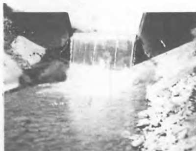
Figure 7 - Trapezoidal Weir Drop in Kittitas North Branch Canal Lateral 17.7
