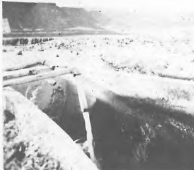
Vents at Inlet to Siphon
