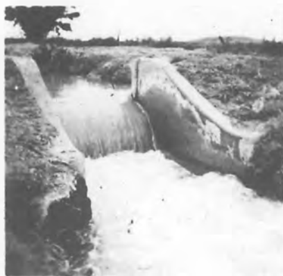
Figure 5 - Rectangular Weir Drop in Gem District D-Line
