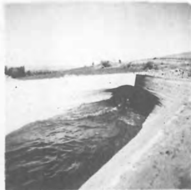
Figure 20 - Entrance to Weed-Swallower Siphon on Tieton Canal
