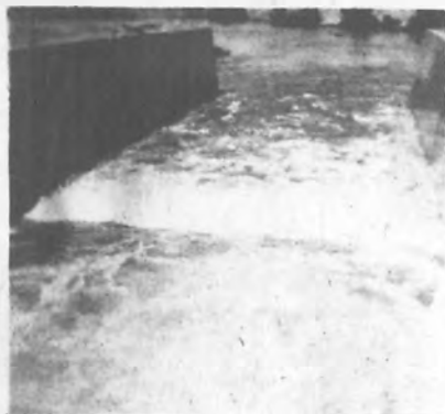
All Gates One-quarter Open. Discharge Approx. 650 Second-Feet
