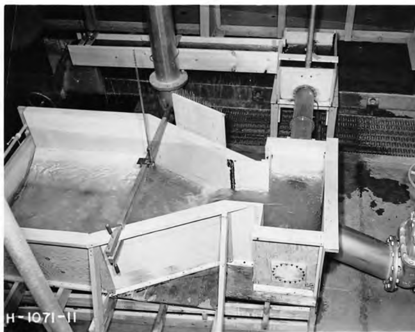
(B) Over-all View with Tee-shaped Forebay--60 cfs Total Discharge with Right Outlet Operating
