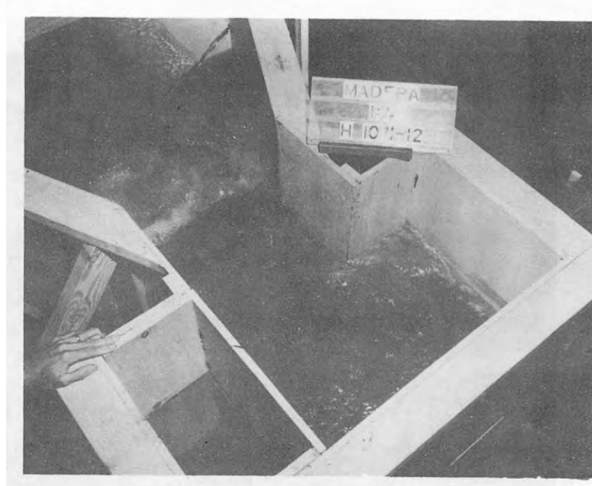
(A) Tee-Shaped Forebay--60 cfs Total Discharge with Right Turnout Operating
