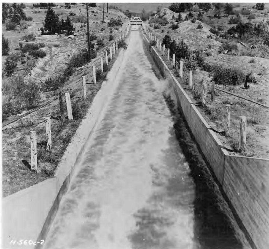
B. Wave in upper section of wasteway caused by entrance condition. Discharge 922 second-feet.
