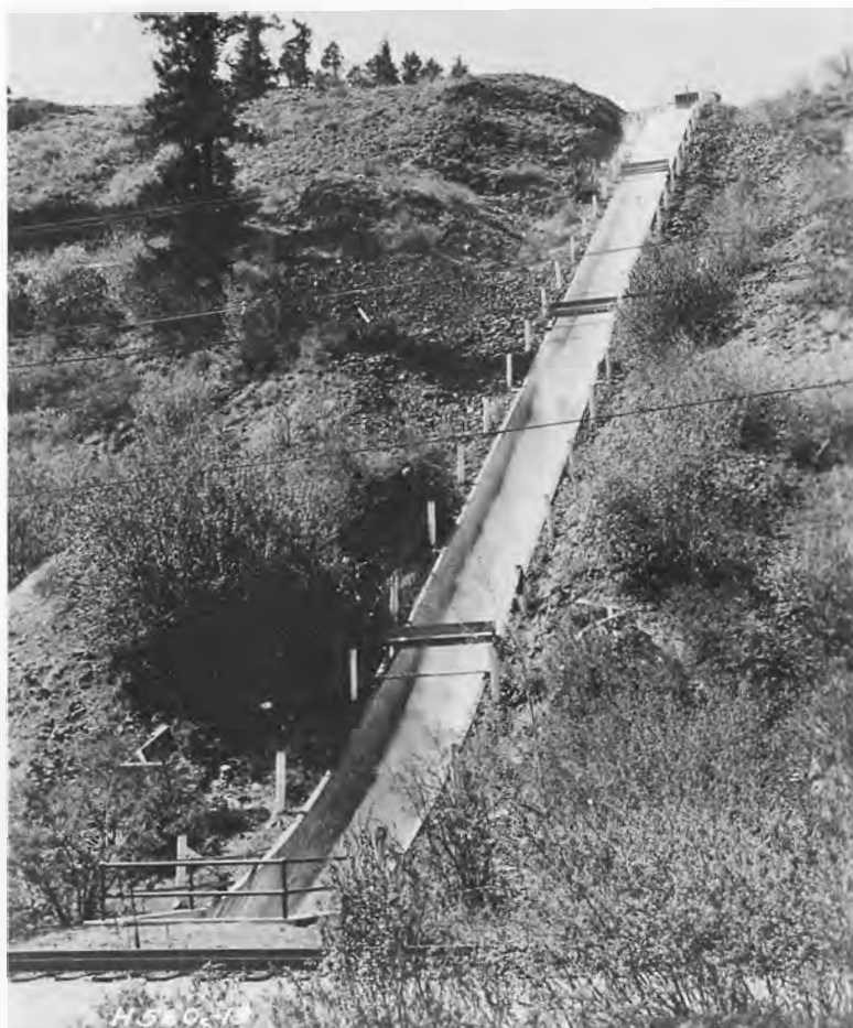
B. Flow conditions on 33°-10' slope. Discharge 922 second-feet
