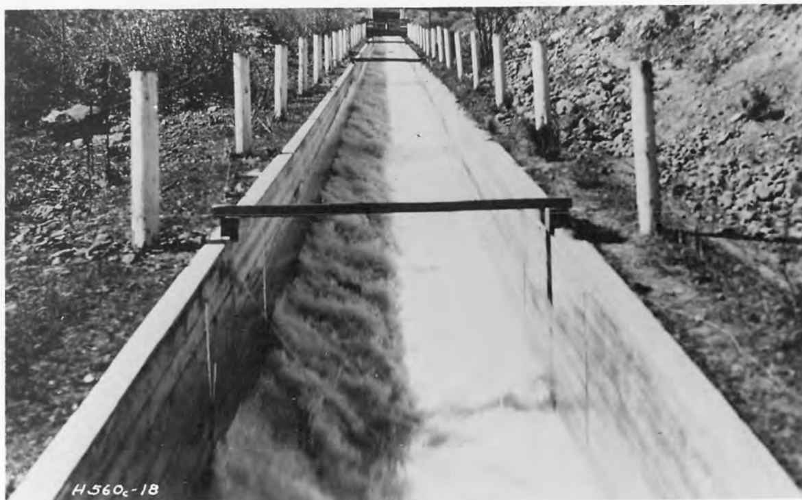
A. Flow conditions on 10°-12' slope. Discharge 777 second-feet.
