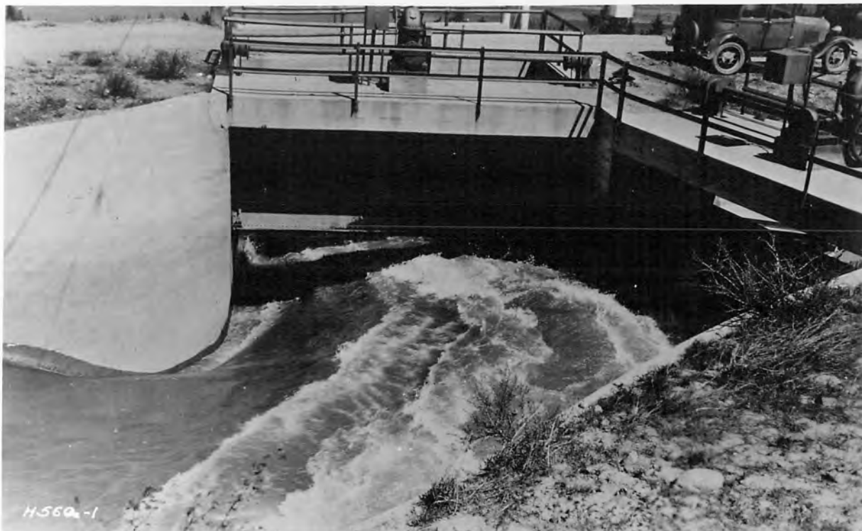
A. Wasteway entrance. Discharge 922 second-feet.
