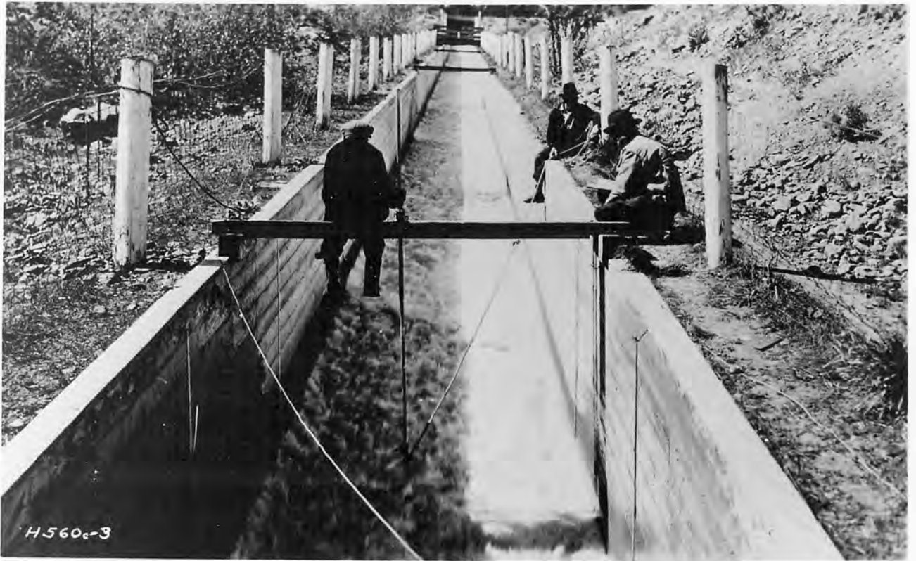
A. Point gage used for obtaining depth of flow.
