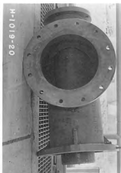
E. Outlet of main absorber at point where orifice for stage 3 is attached. Stage 2 is at bottom of photo.
