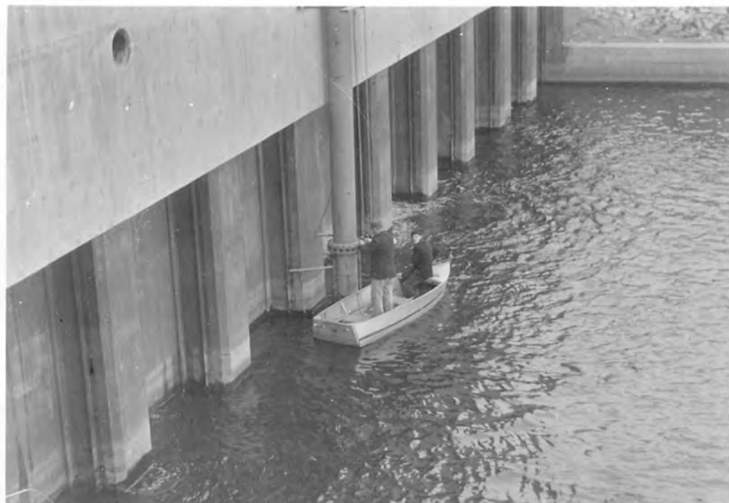
B. Repairing butterfly valve from rowboat.
