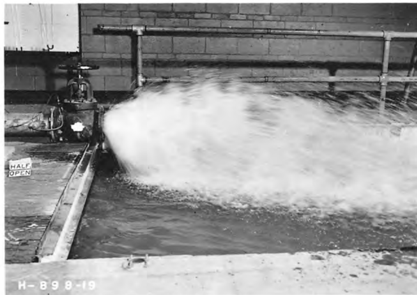
A. Valve open 1/2 of stem travel.
