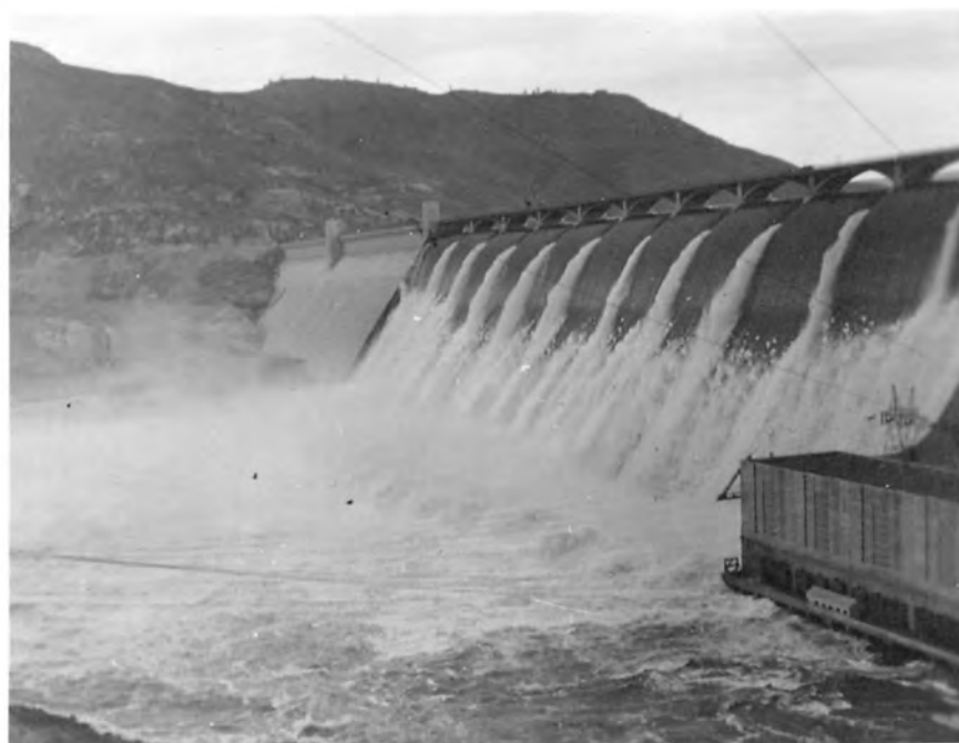
B. Grand Coulee Dam operating at a discharge of 570,000 second feet
