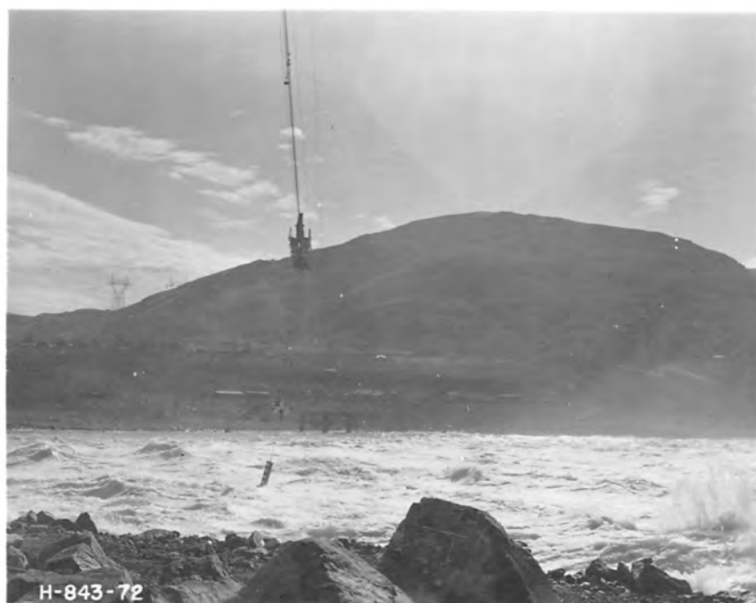
B. Movement of pile hammer by forces exerted by waves and water velocity - River Flow 346,000 cfs
