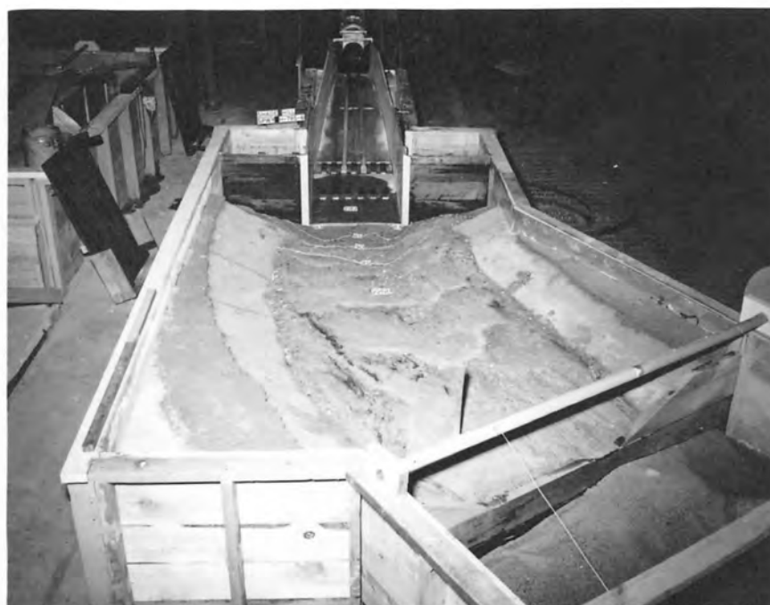
A. Operation at 5,000 second-feet Tailwater elevation 2204.5
