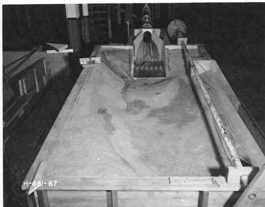
B. Scour after 1/2 hour at 5,600 second-feet T.W. 2012
