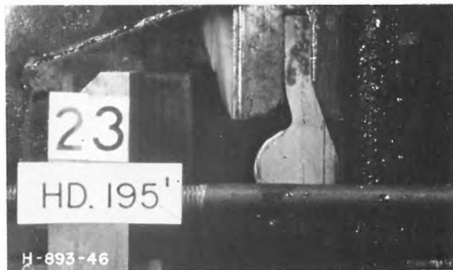
B. Bulb in position for snap-over, control at edge of stem clamp plate.
