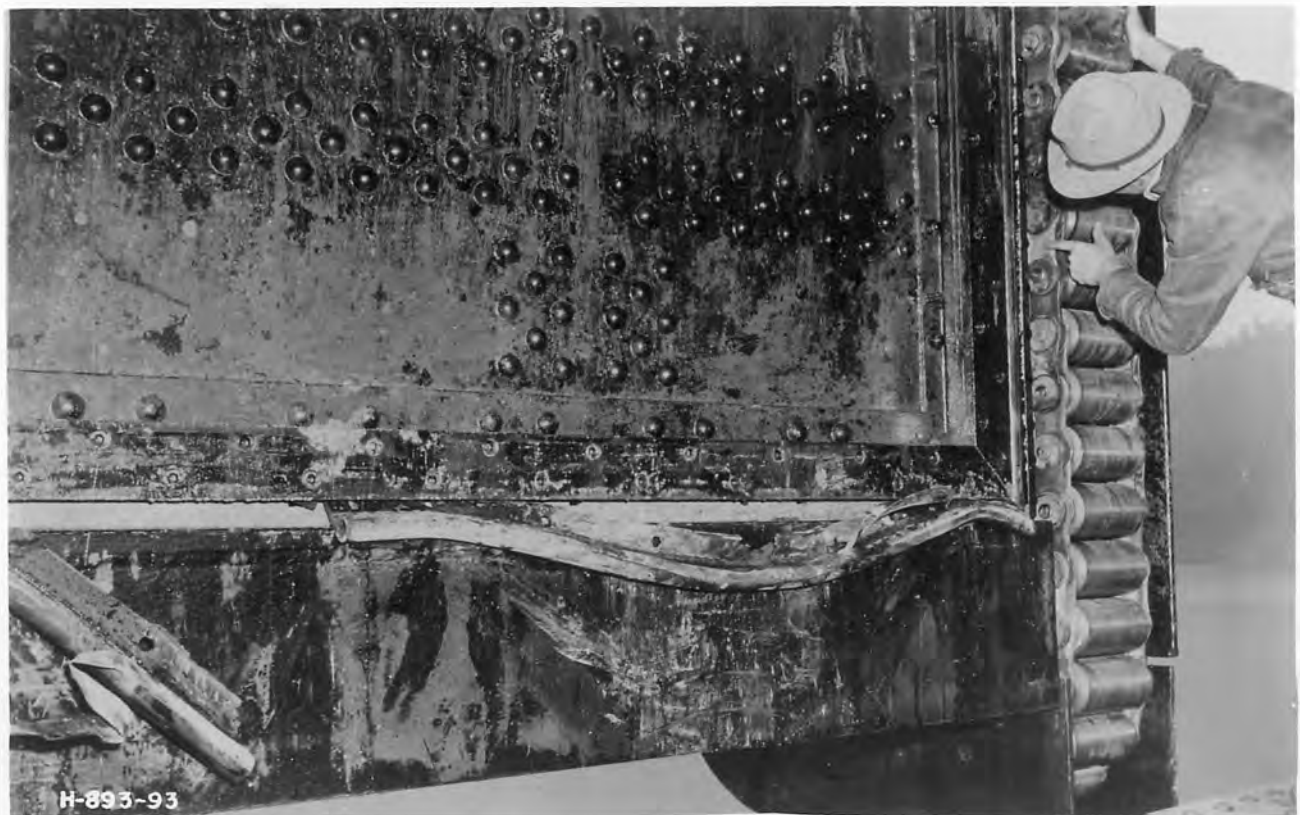
B. East portion of damaged seal shown in Figure 5.
