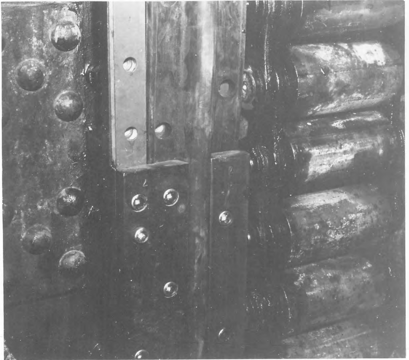
The R-6 coaster gate which was formerly installed in L-3 and was furnished under Specifications No. 905, showing installation of the experimental seal (Reference Drawing No. 222-D-15067). This view of the seal was taken of the upper right hand side of the gate. September 13, 1950.
