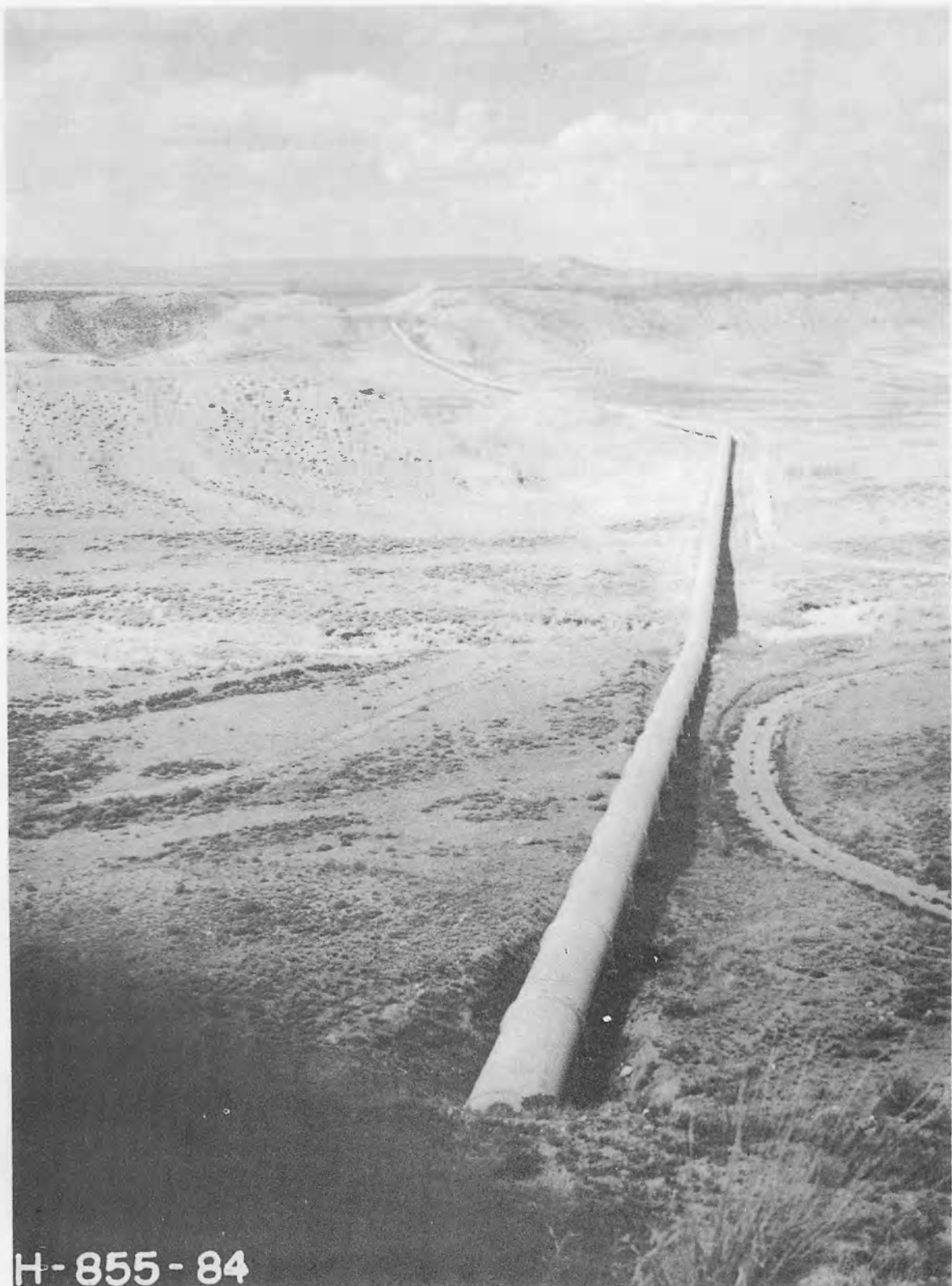
FIGURE 2 Inverted siphon crossing creek valley. Tube is of steel having a 104-inch Internal Diameter, and approximate length of 3500 feet.
