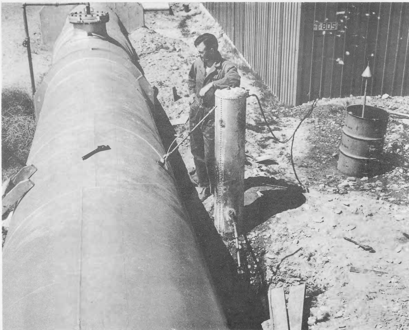
FIGURE 7 Brine tank and injection equipment on 60-inch steel pump discharge line approximately 1500 feet long.
