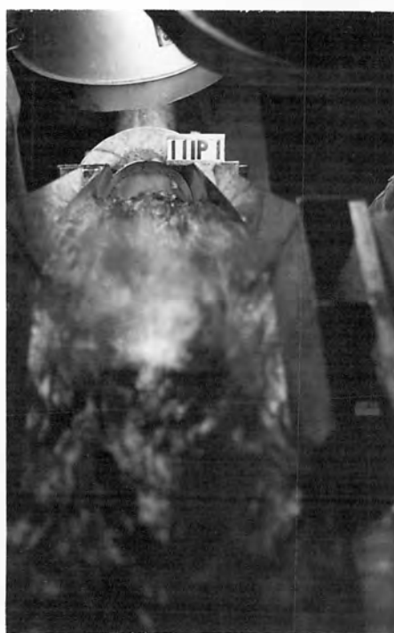
D. LOOKING DOWN CHUTE WITH DISCHARGE 5,000 SECOND-FEET
