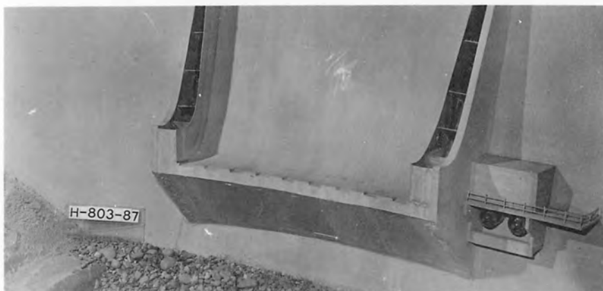
C. Drain slots alternate with equal widths of normal bucket profile to form dentated lip. Outlet works is at side of bucket.
