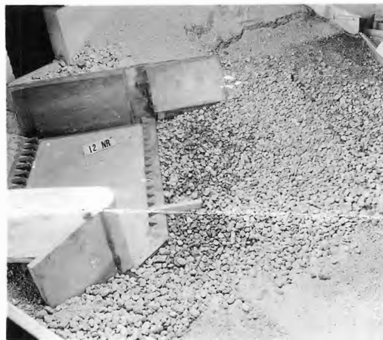
(C) POOL AND RIPRAP AFTER FINAL TESTS
