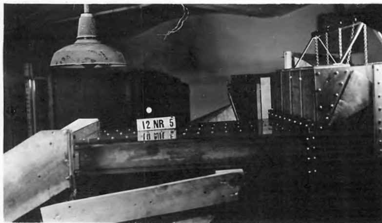
(C) CULVERTS AND WASTEWAY GATES
