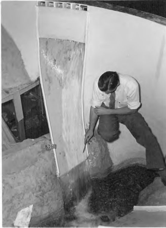
A. Flow concentrated. Gate 1 open.
