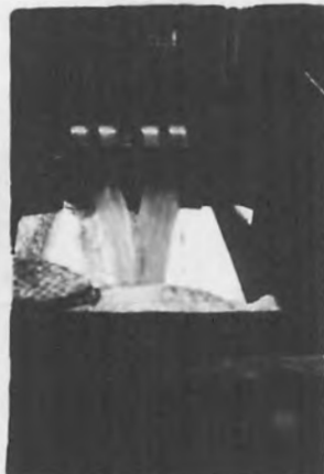
F. GATES THREE-FOURTHS OPEN LEFT TUNNEL FULL RIGHT TUNNEL FREE
