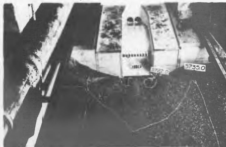
D. EROSION OF RIVER BED AFTER ONE HOUR RUN
