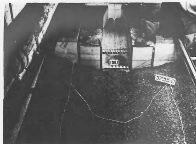
B. EROSION OF RIVER BED AFTER ONE HOUR RUN DISCHARGE 4000 SECOND-FOOT
