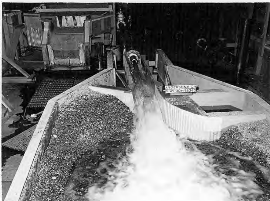
A. Flow conditions in diversion and river channels with valve discharge of 4210 cfs.
