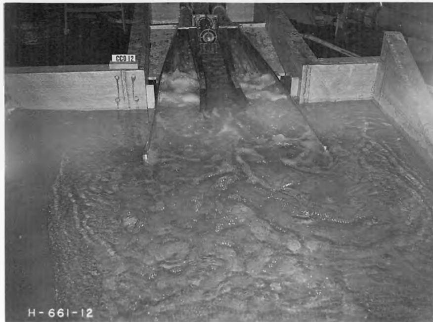
A. Both outside conduits operating - 6,000 second-feet
