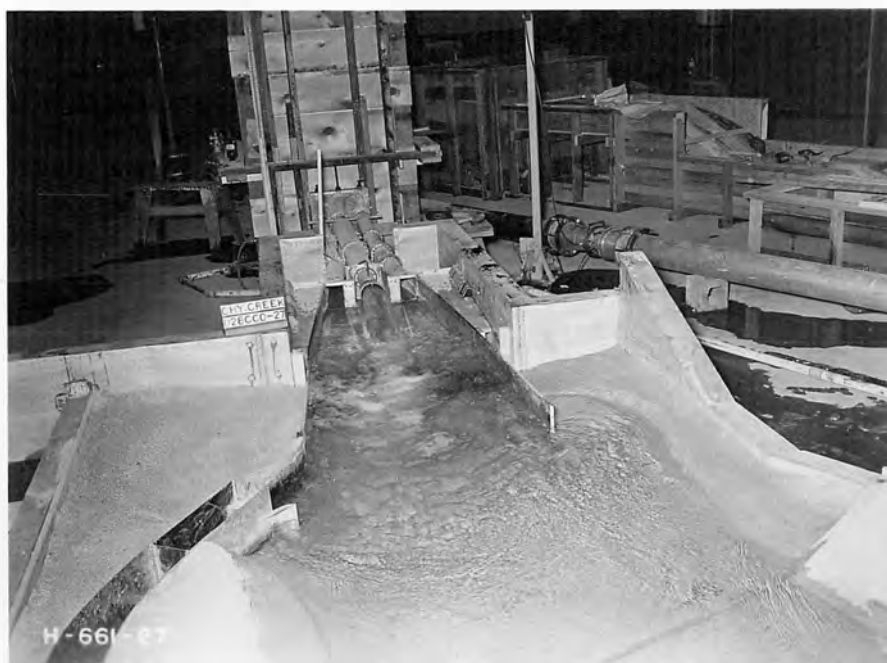
B. Hollow-jet valve operating - 1,500 second-feet. Flow is to the right of basin centerline.
