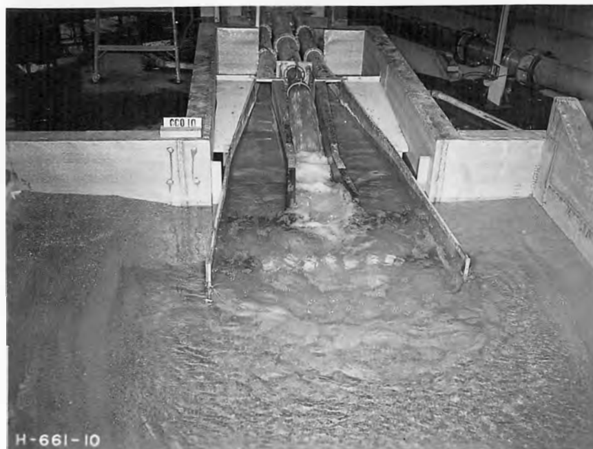
A. Hollow-jet valve discharging 1,500 second-feet
