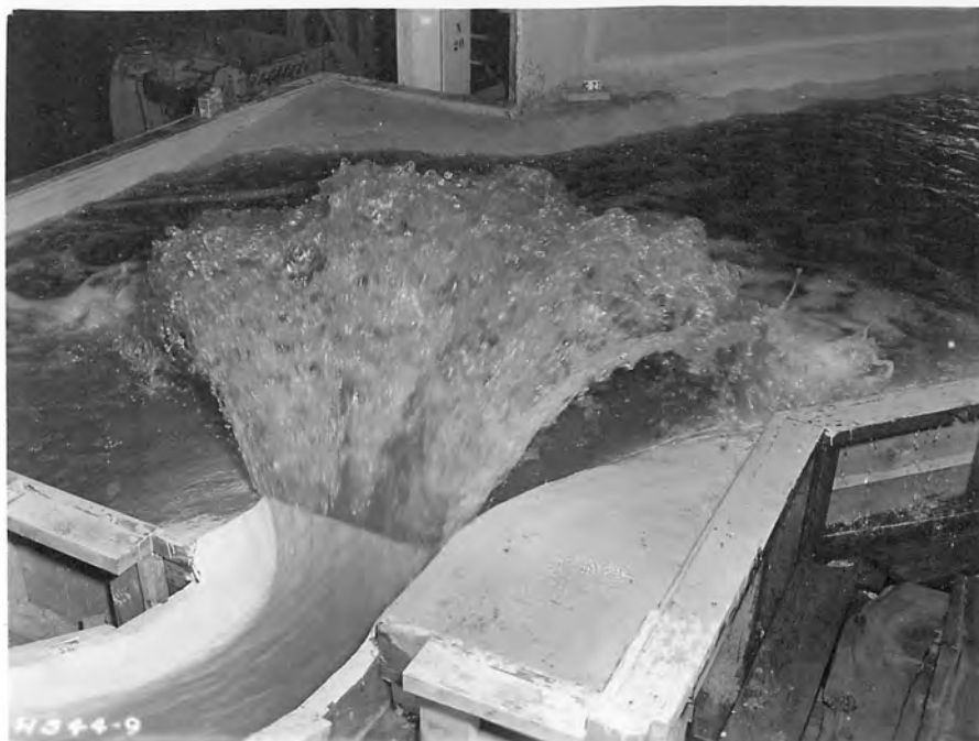
A. Diffuser Bucket Discharging 10,000 Second-feet.
