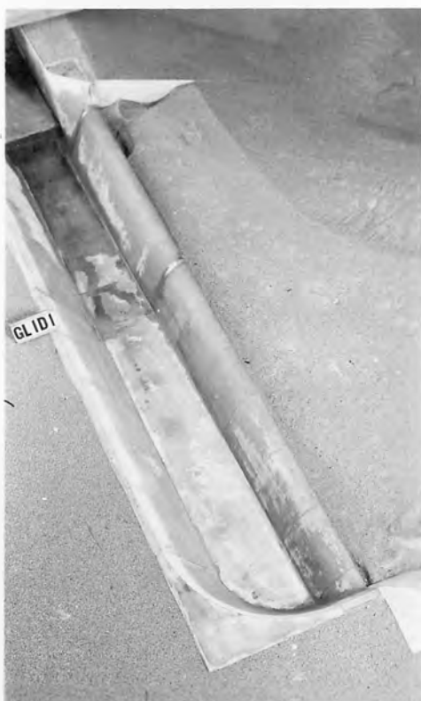
C. Erosion caused by flow of 12,000 second-feet.
