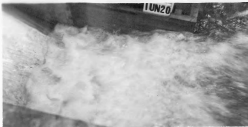
A. Position of hydraulic jump. Tailwater El. 3771.0.
