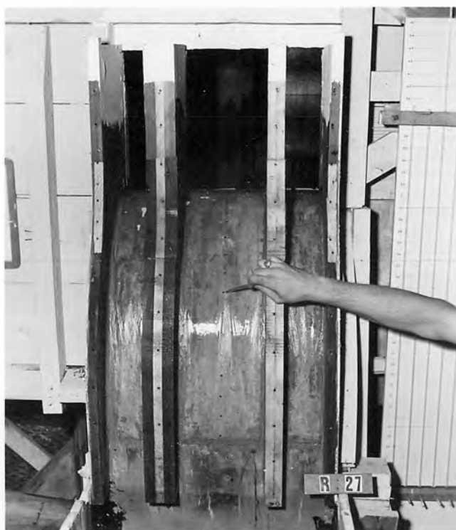
B. Crest shape and piezometers with deflector removed.
