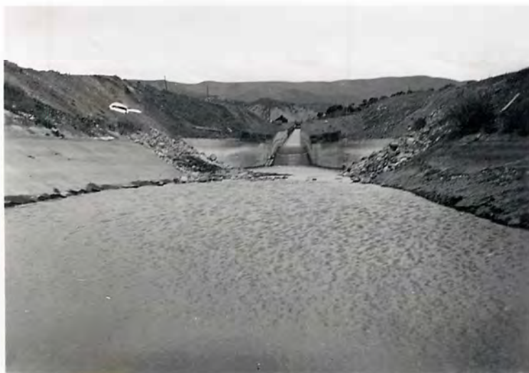
A - Restriction below stilling pool looking upstream
