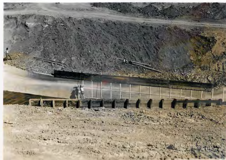
D - Painting grid lines on wall of stilling pool
