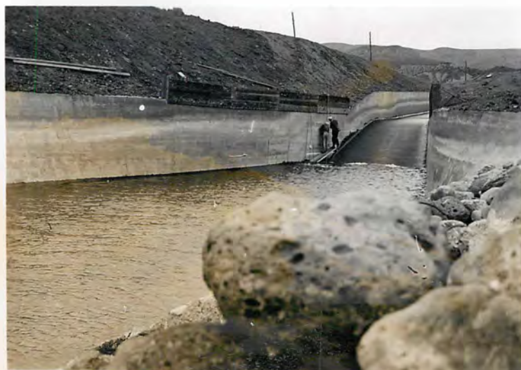
C - Painting grid lines on wall of stilling pool
