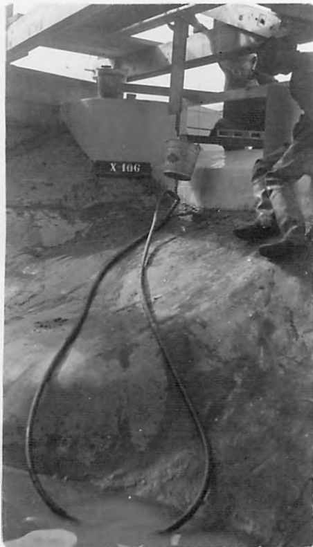
A-METHOD OF OBSERVING CREST ELEVATIONS
