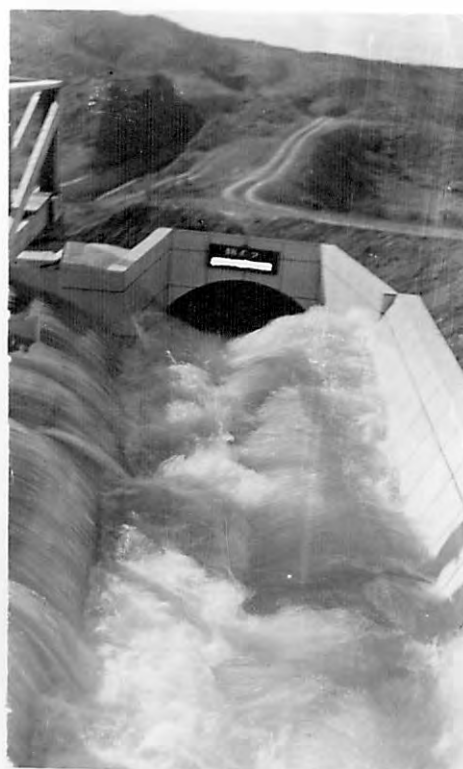
C-DISCHARGE 144,000 SEC. FT. LARGEST FLOW FROM DOWNSTREAM GATES
