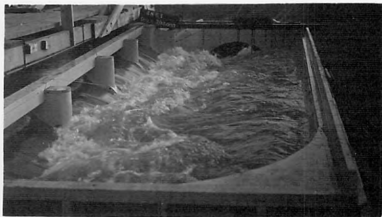
CONDITIONS WITH CROSS WEIR LOWERED 12 FT.
