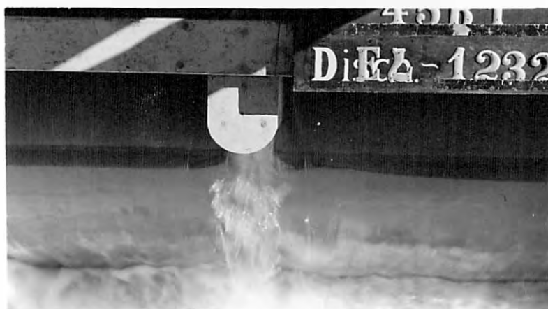
GATES RAISED \frac{3}{4} -DISCHARGE 90,000 SEC FT
