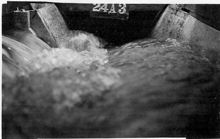
A-15 FT. WEIR AT END OF CHANNEL
