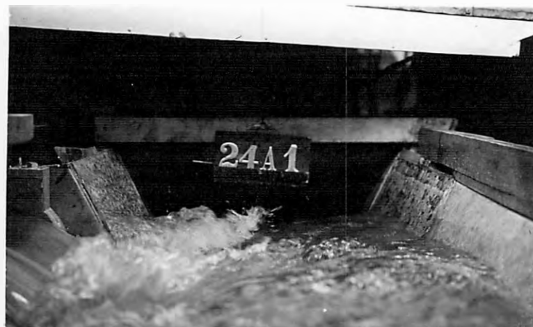
C-30 FT. WEIR AT END OF CHANNEL
