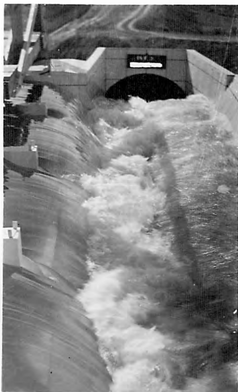
B-DISCHARGE 144,000 SEC. FT. LARGEST FLOW FROM UPSTREAM GATES
