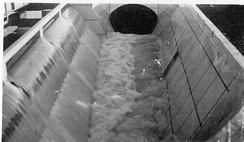
A-DISCHARGE 31,500 SEC. FT. ALL GATE CRESTS AT EL. 1221.7
