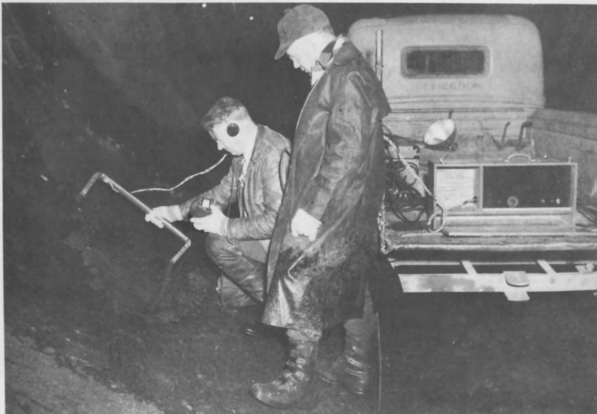
AD7-2 - ELECTRONIC DETECTOR - Use of a decibel meter instead of headphones with the electronic detector, as shown, is believed by the operator to be more satisfactory in the noisy tunnel. L. R. Murphy
