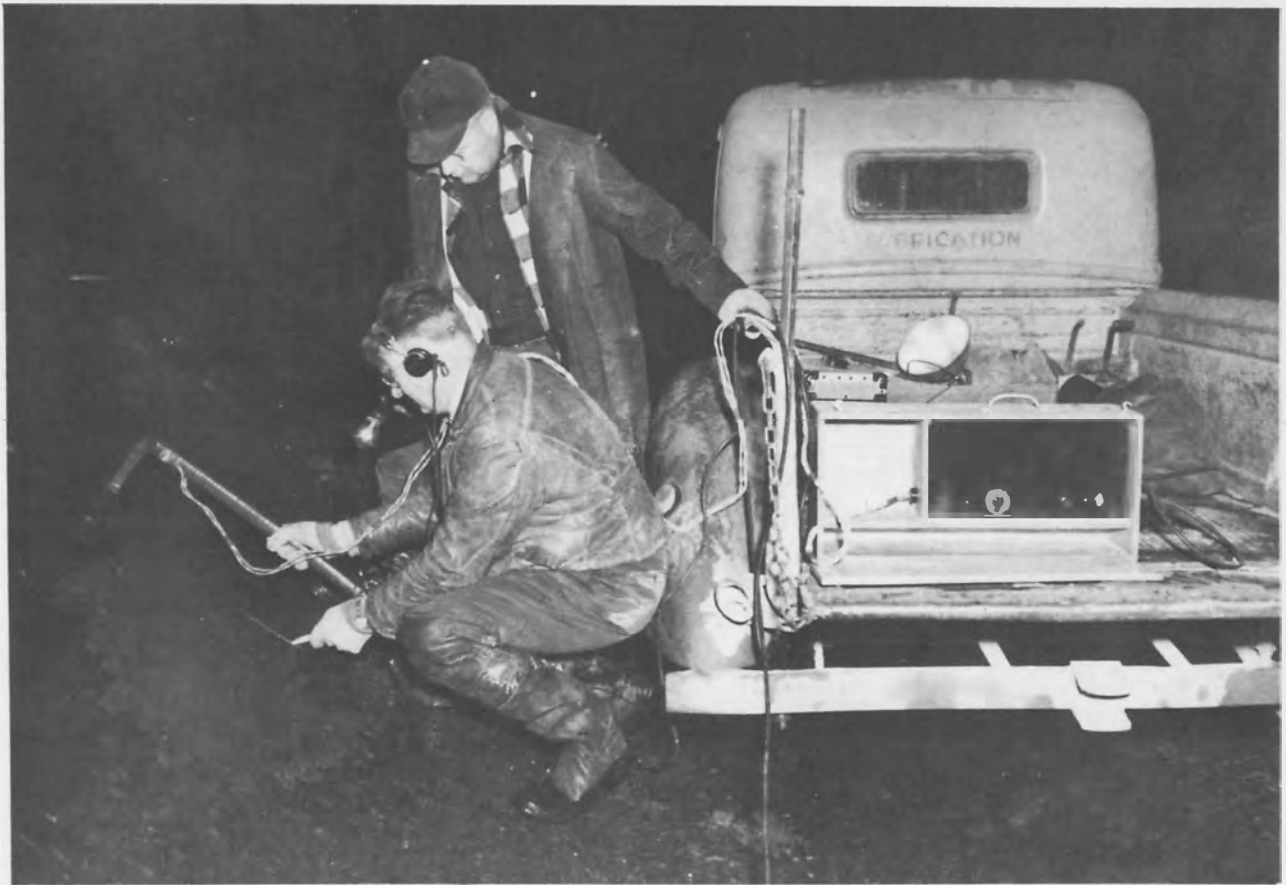
3702 - ELECTRONIC DETECTOR - Inspectors A. V. Lane and C. A. Jungquist are operating the electronic detector to accurately determine the location of imbedded reinforcement in the outlet tunnel concrete lining, and thereby determining locations for drilling grout holes. L. R. Murphy
