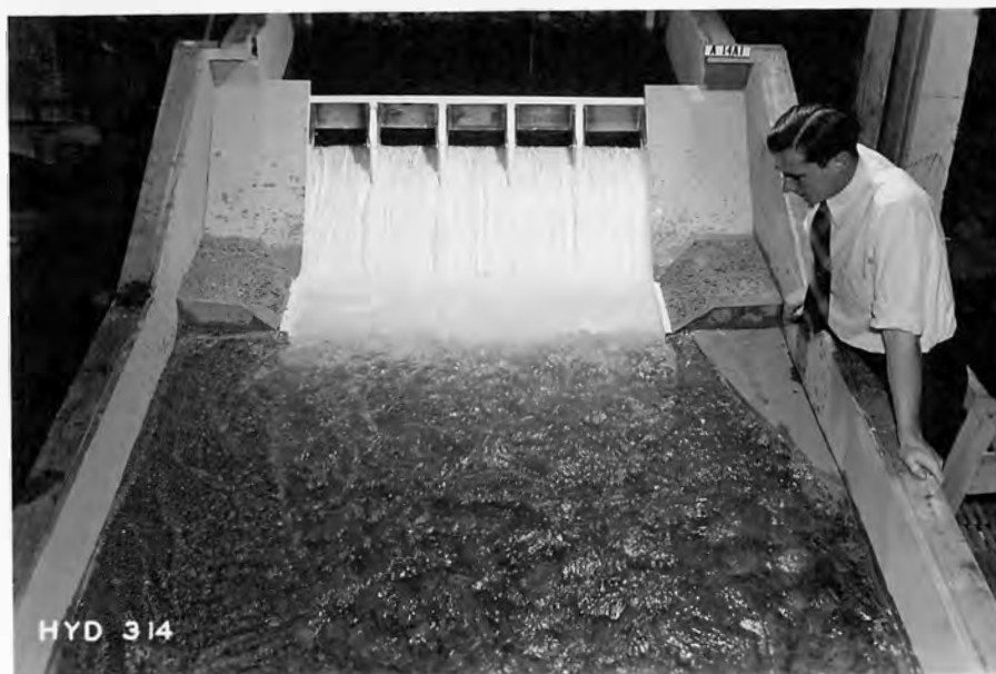
A - Flow of 50,000 second-feet over spillway.
