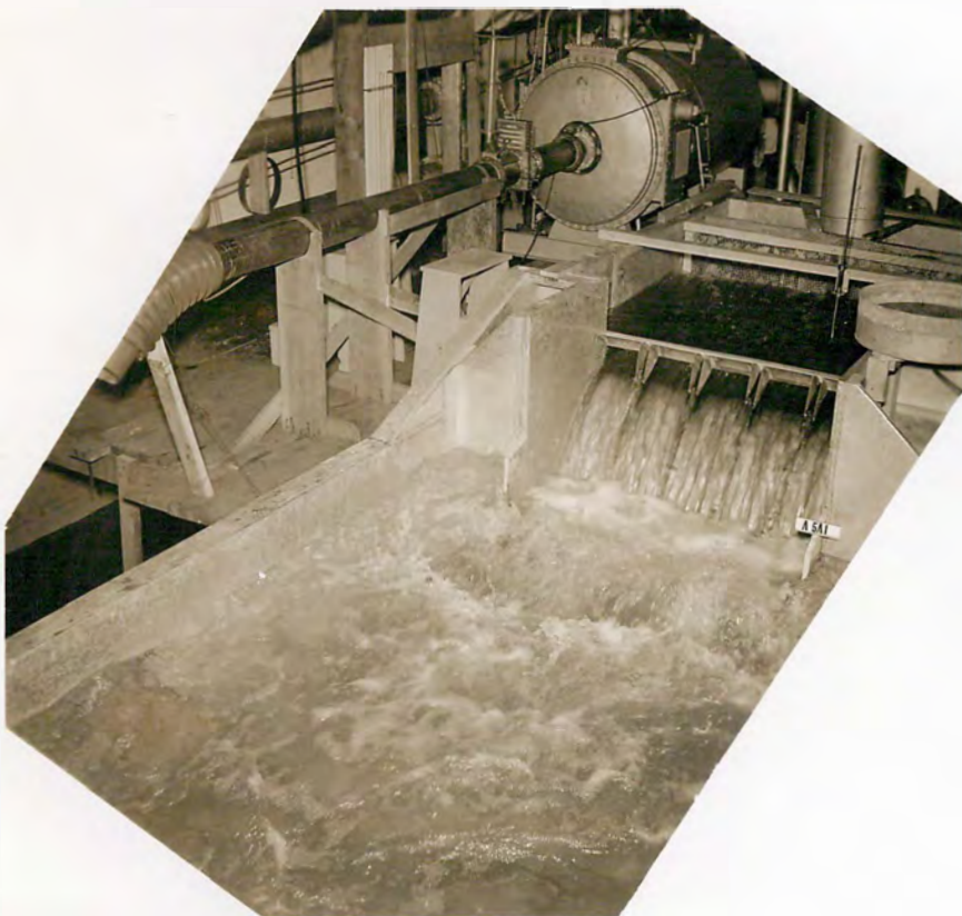
A - Flow of 277,000 second-feet over spillway.
