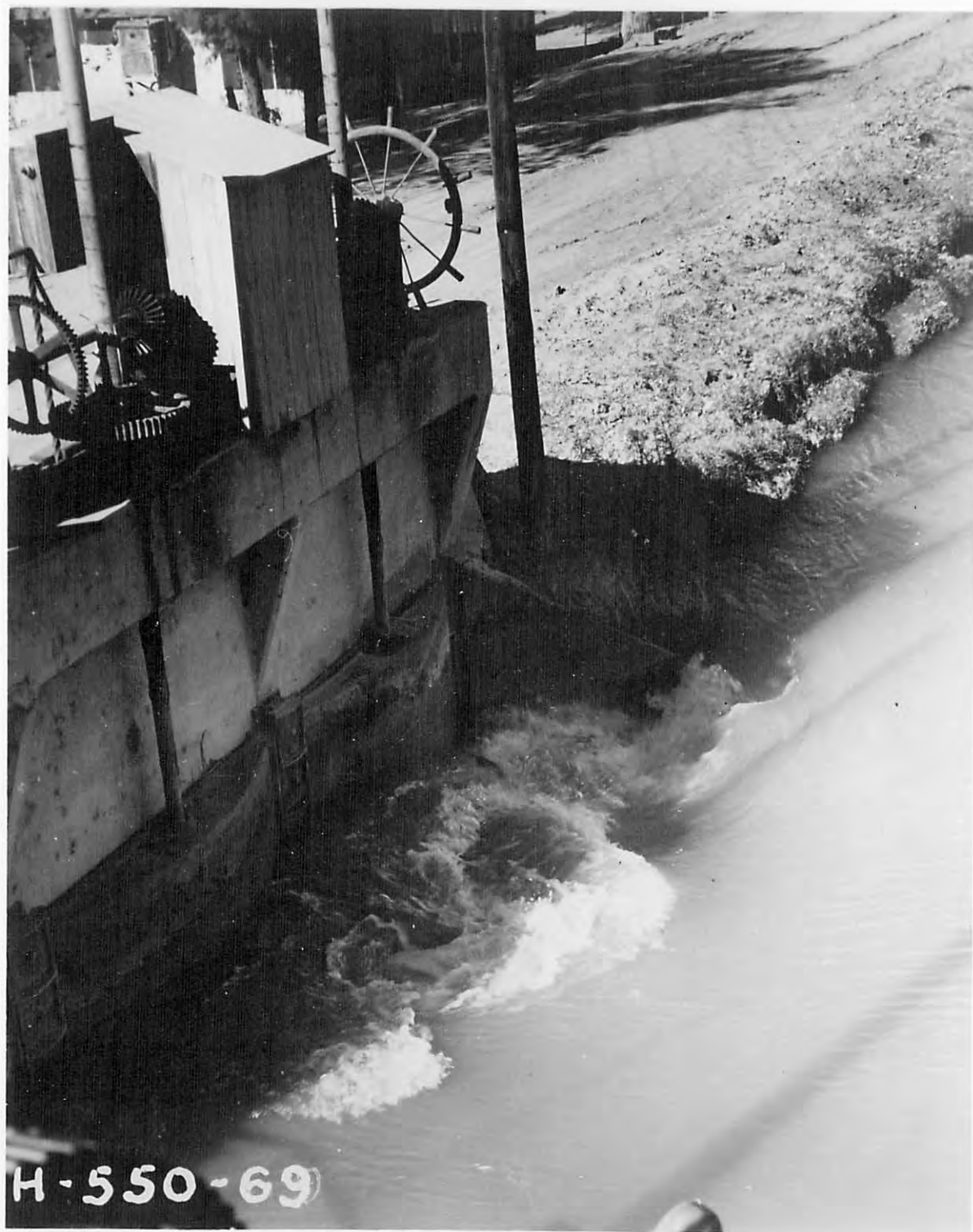
Entrance Conditions at Upstream End of Structure--Discharge Approximately 1600 Second-feet. January 16, 1947.
