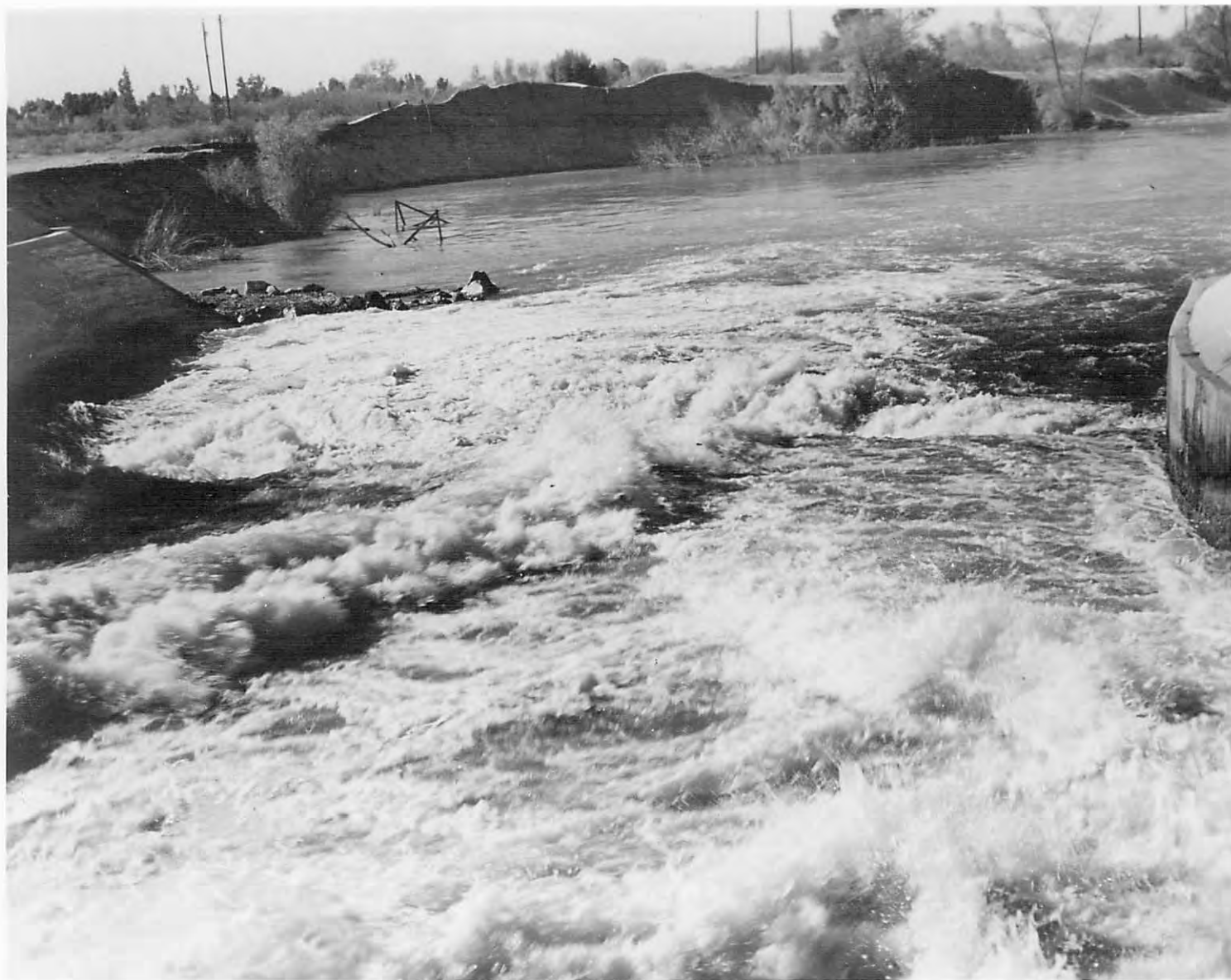
Chute and Pool Conditions--Discharge Approximately 1600 Second-feet. January 16, 1947. California Wasteway--Yuma Project--Arizona, California.
