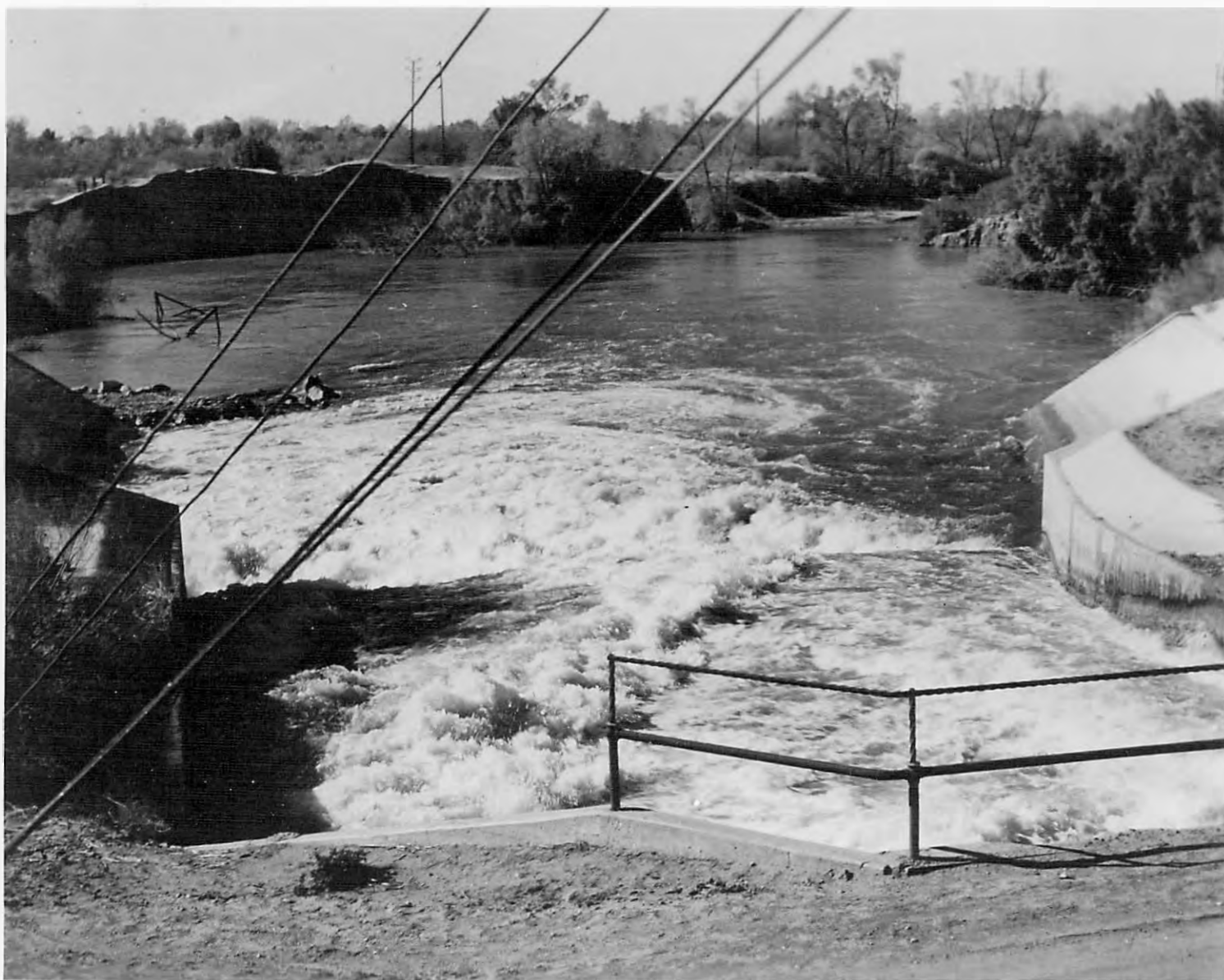
Chute and Pool Conditions--Discharge Approximately 1600 Second-feet. January 16, 1947. California Wasteway--Yuma Project--Arizona, California.
