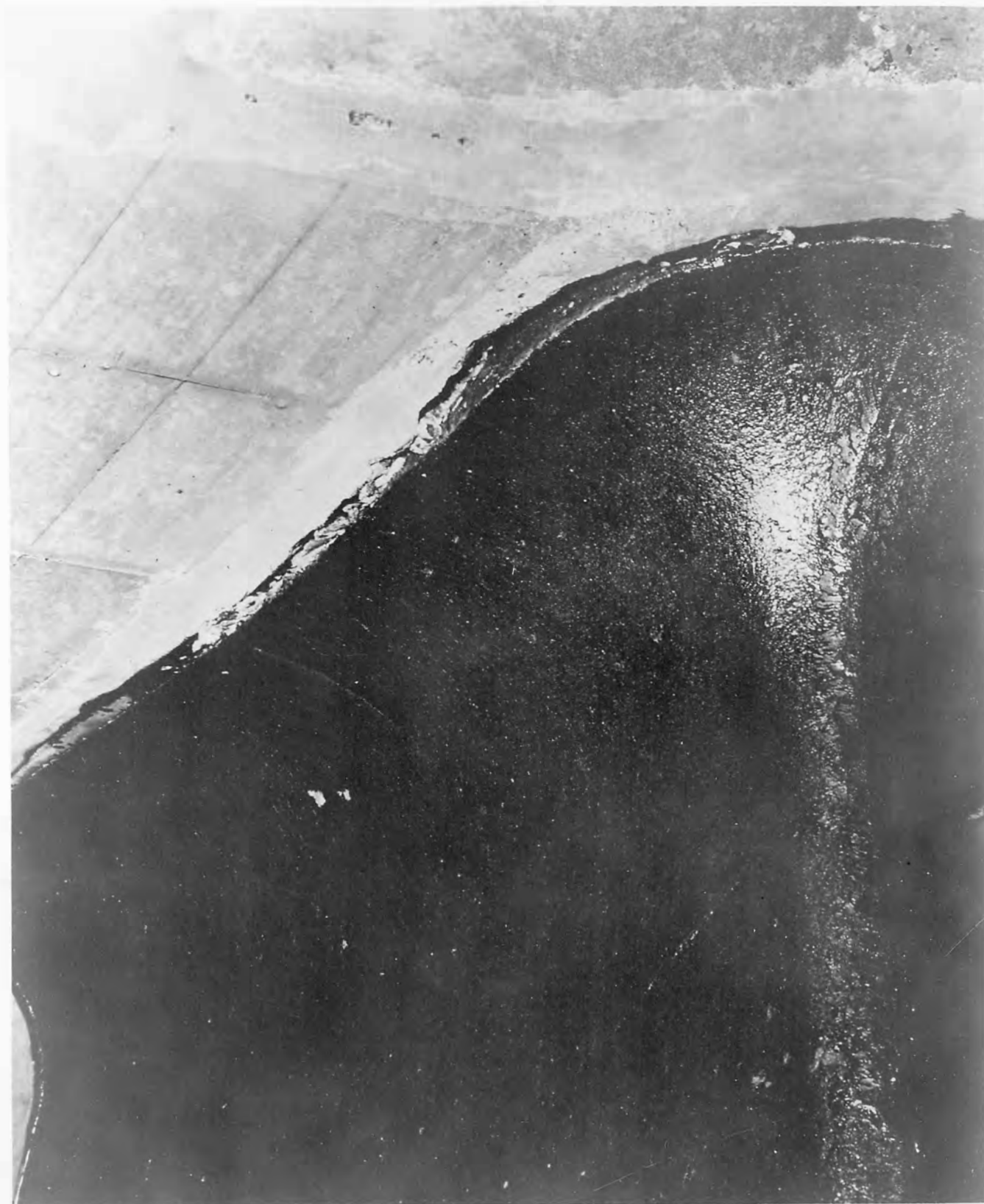
Photograph 13248-3, August 10, 1945: View from draft tube floor showing chipped edge in concrete adjacent to top of metal pier nose, left pier of draft tube R-9 outlet operated at full capacity for approximately 23 hours.
