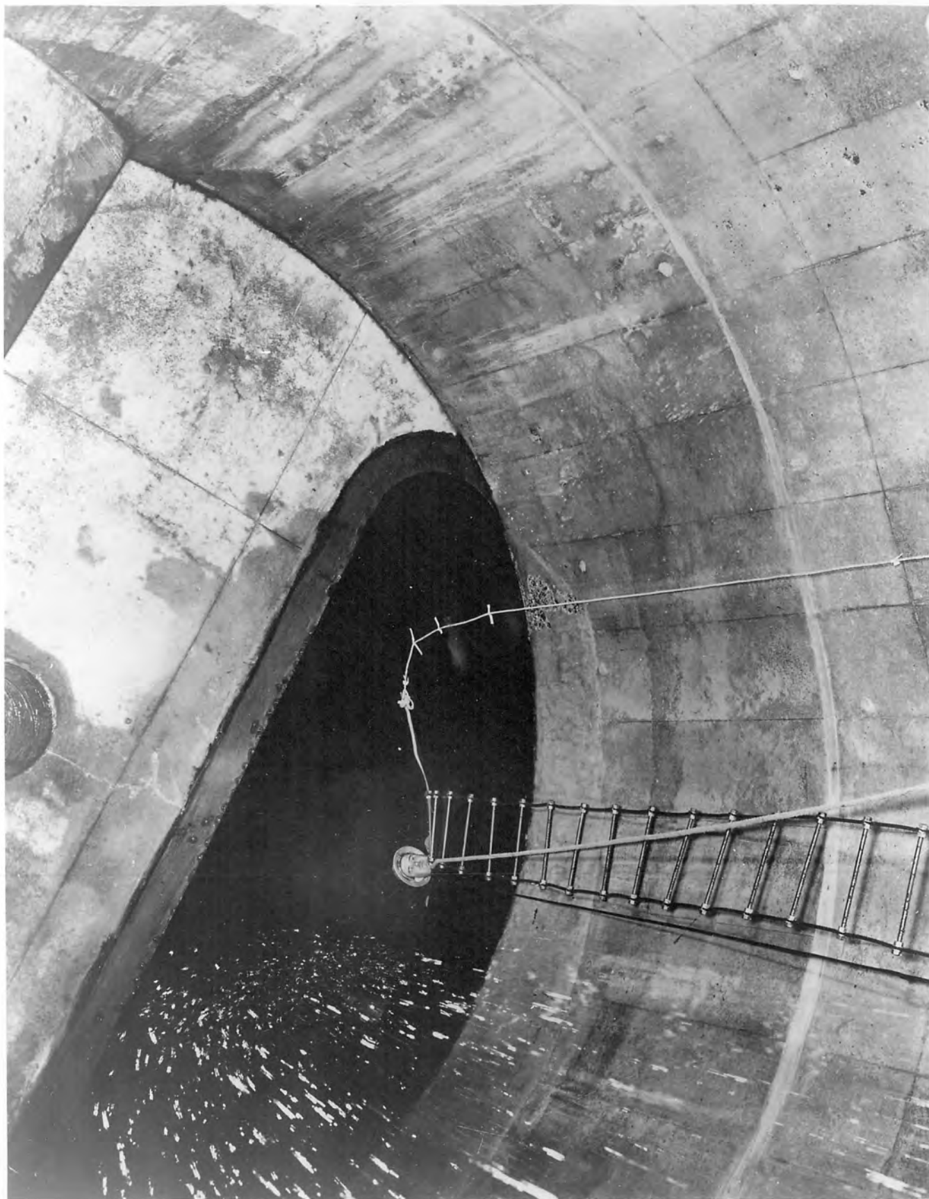
Fig. 3. Photograph 13044-3, June 7, 1945: View from floor of draft tube showing pitting by cavitation in the inner curve at the left side of the steel elbow and in the wall of the anchor block immediately below, after operation of the R-9 outlet for tests on May 25 and June 5, 1945. Discontinuities in flow boundary accentuated by small rope passing over damaged areas.
