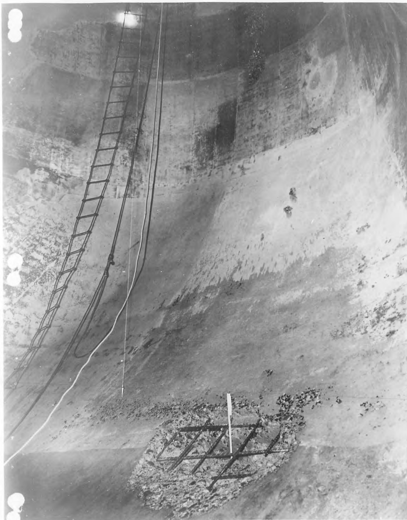
Photograph 13246-3, August 10, 1945: View from draft tube floor showing extent of cavitation in wall of anchor block and in floor of draft tube in vicinity of recess from which patch was torn during first six hours of operation, after operation of the R-9 outlet for approximately 23 hours on August 7, 8, and 9, 1945. Plumb bob indicates centerline of 18-inch vent in top of anchor block.
