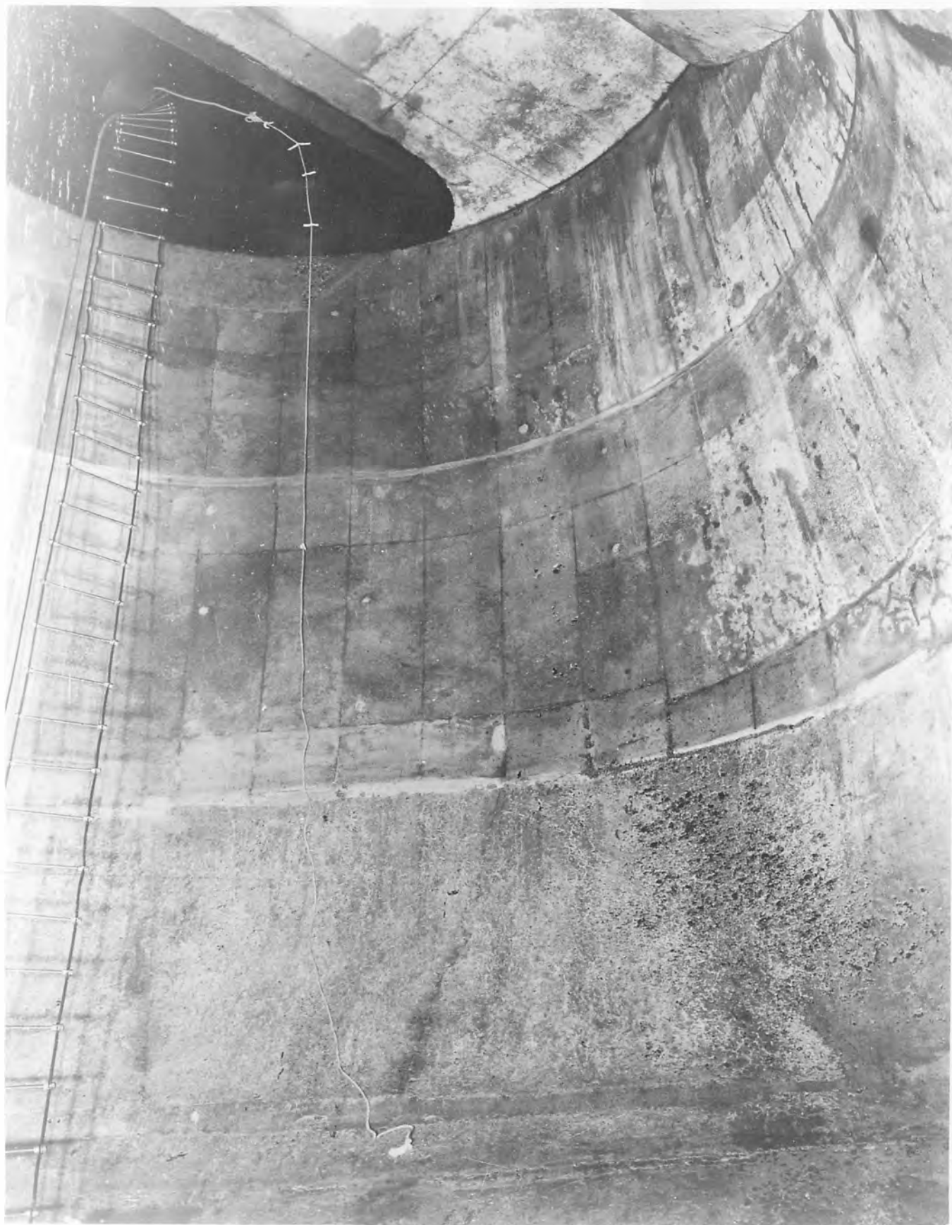
Fig. 5. Photograph 13051-3, June 7, 1945: View from floor of draft tube showing pitting by cavitation in the inner curve at the left side of the steel elbow and in the wall of the anchor block and draft tube directly downstream, after operation of the R-9 outlet for tests on May 25 and June 5, 1945.
