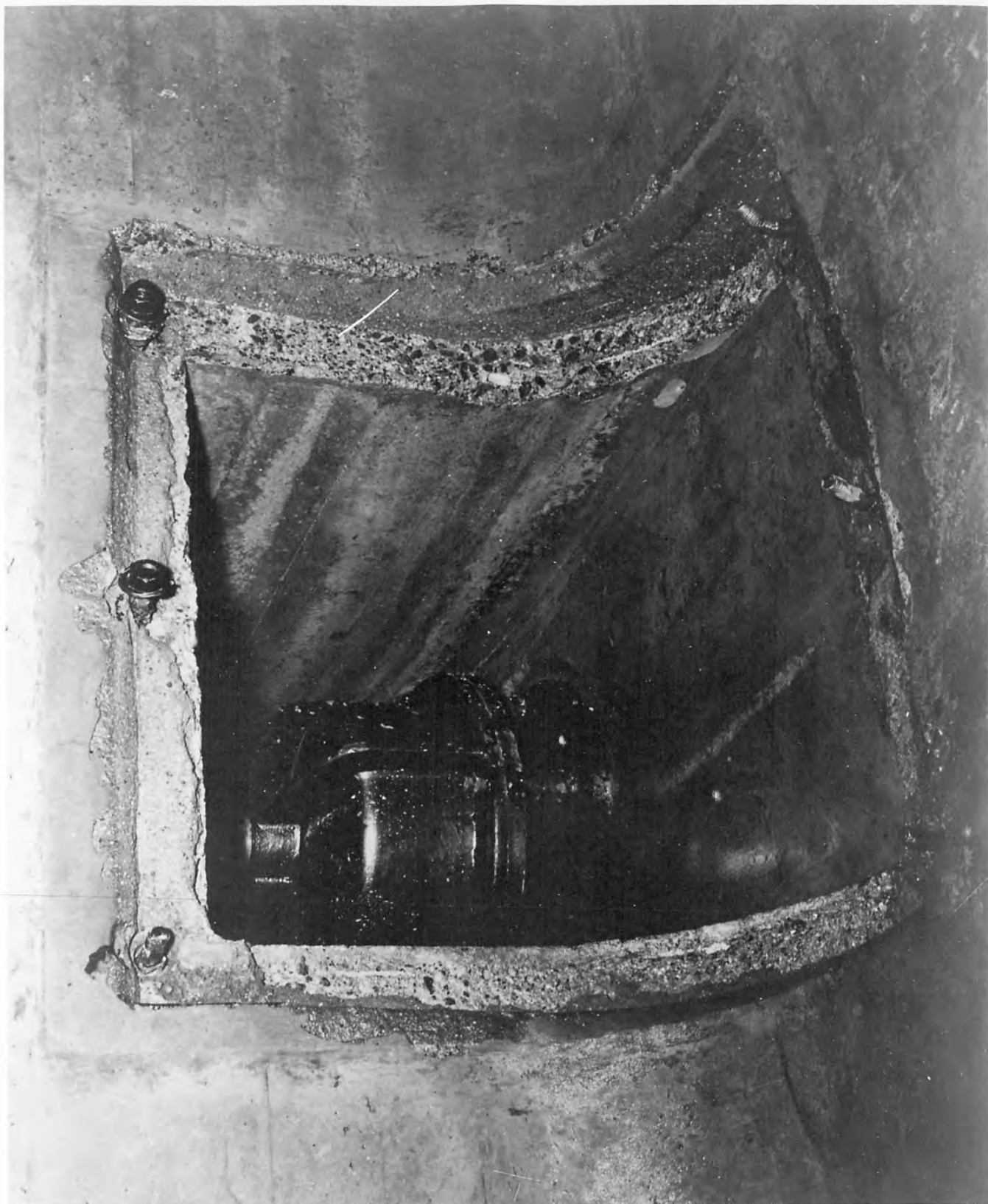
Photograph 13249-3, August 10, 1945: View from draft tube floor showing recess from which grating to draft tube drain valves was torn during operation of the R-9 outlet at full capacity for approximately 23 hours on August 7, 8 and 9, 1945.
