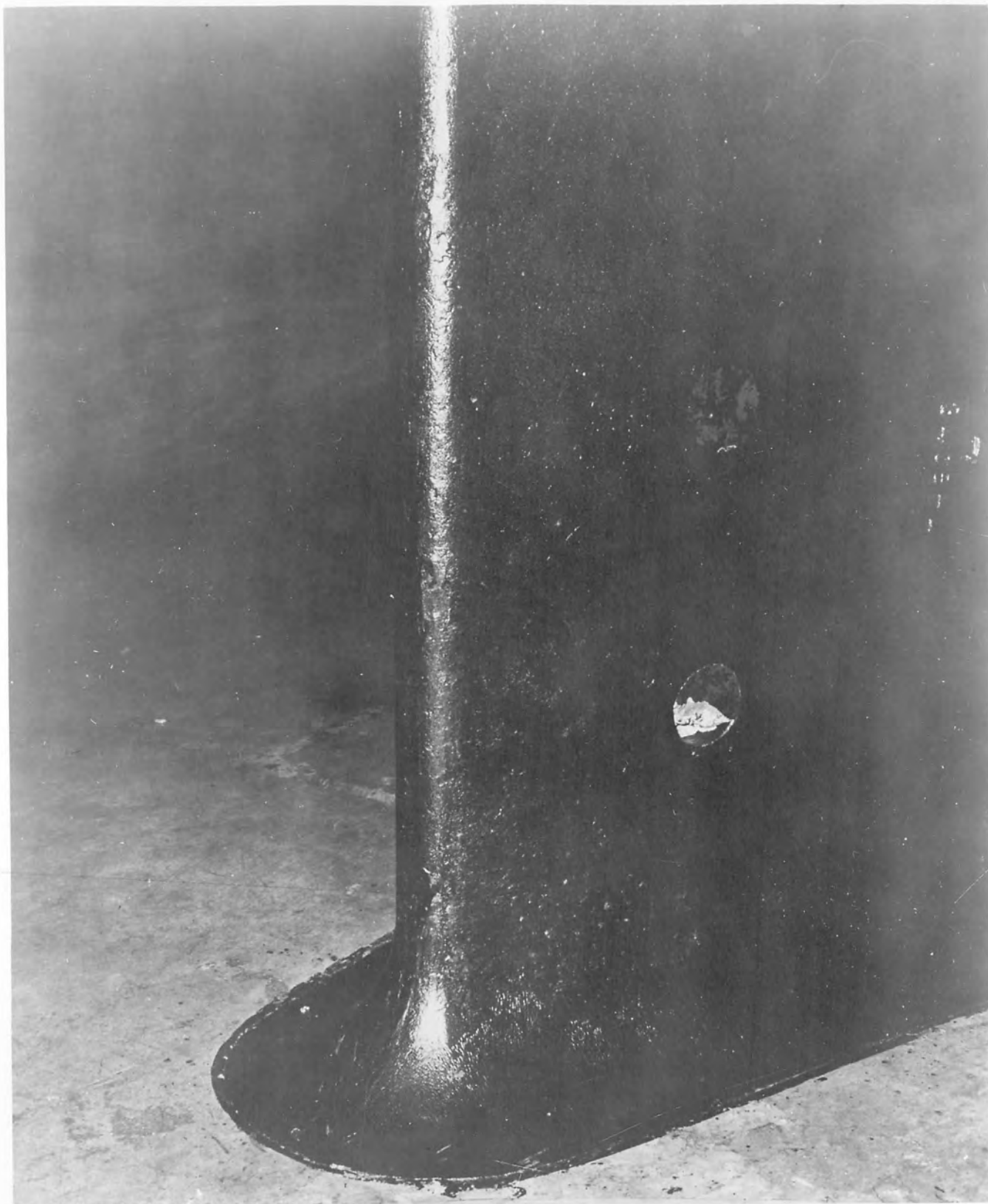
Photograph 13250-3, August 10, 1945: View from draft tube floor showing hole in right side of the right draft tube pier nose from which part of concrete is missing after operation of the R-9 outlet at full capacity for approximately 23 hours on August 7, 8 and 9, 1945.
