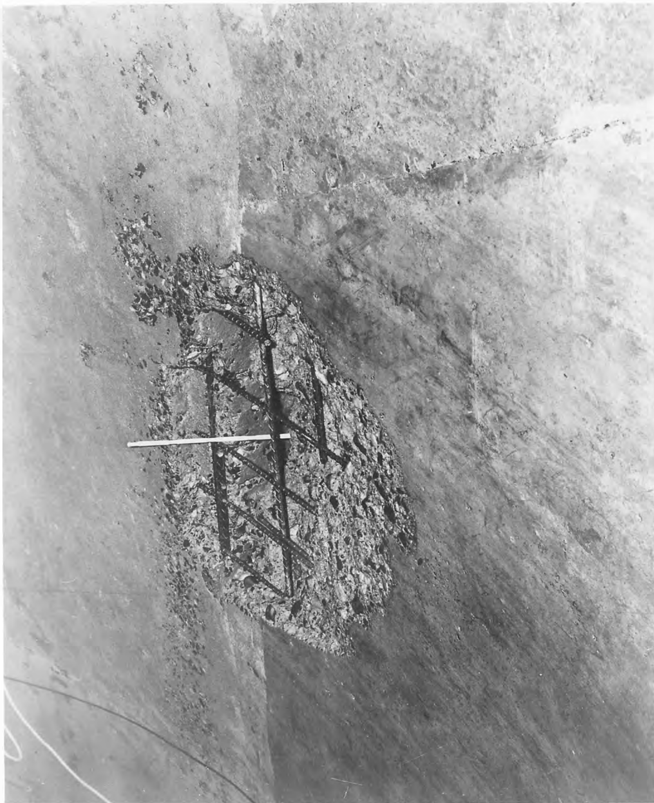
Photograph 13242-3, August 9, 1945: View from draft tube floor showing pitting by cavitation in area near joint 17'-9" upstream from draft tube pier nose from which patch was torn, after operation of the R-9 outlet for approximately 23 hours at full capacity on August 7, 8 and 9, 1945.
