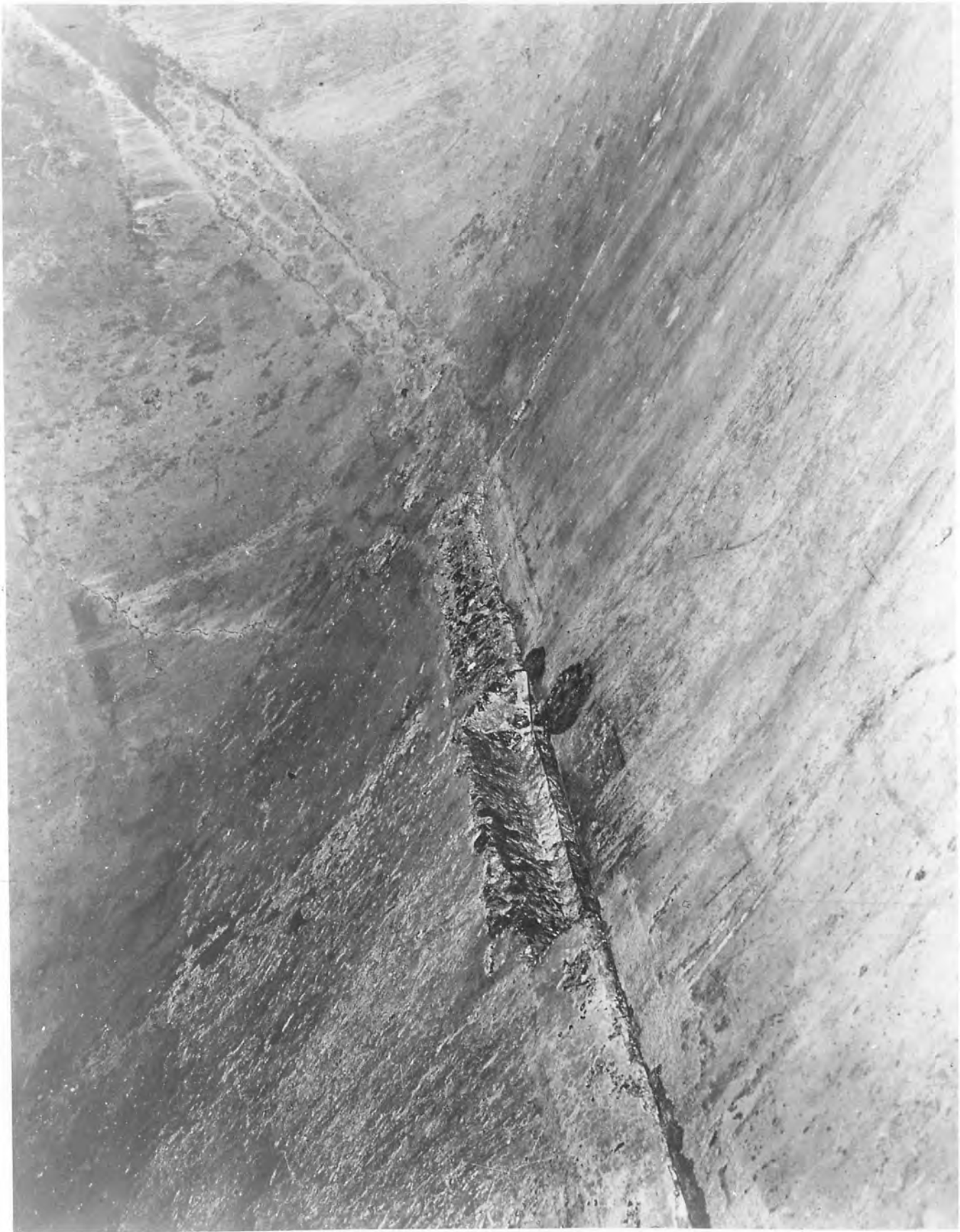
Fig. 6. Photograph 13045-3, June 7, 1945: View from floor of draft tube showing recess in joint upstream from draft tube piers from which patch has been torn by flow from 84-inch needle valve, after operation of the R-9 outlet for tests on May 25 and June 5, 1945.
