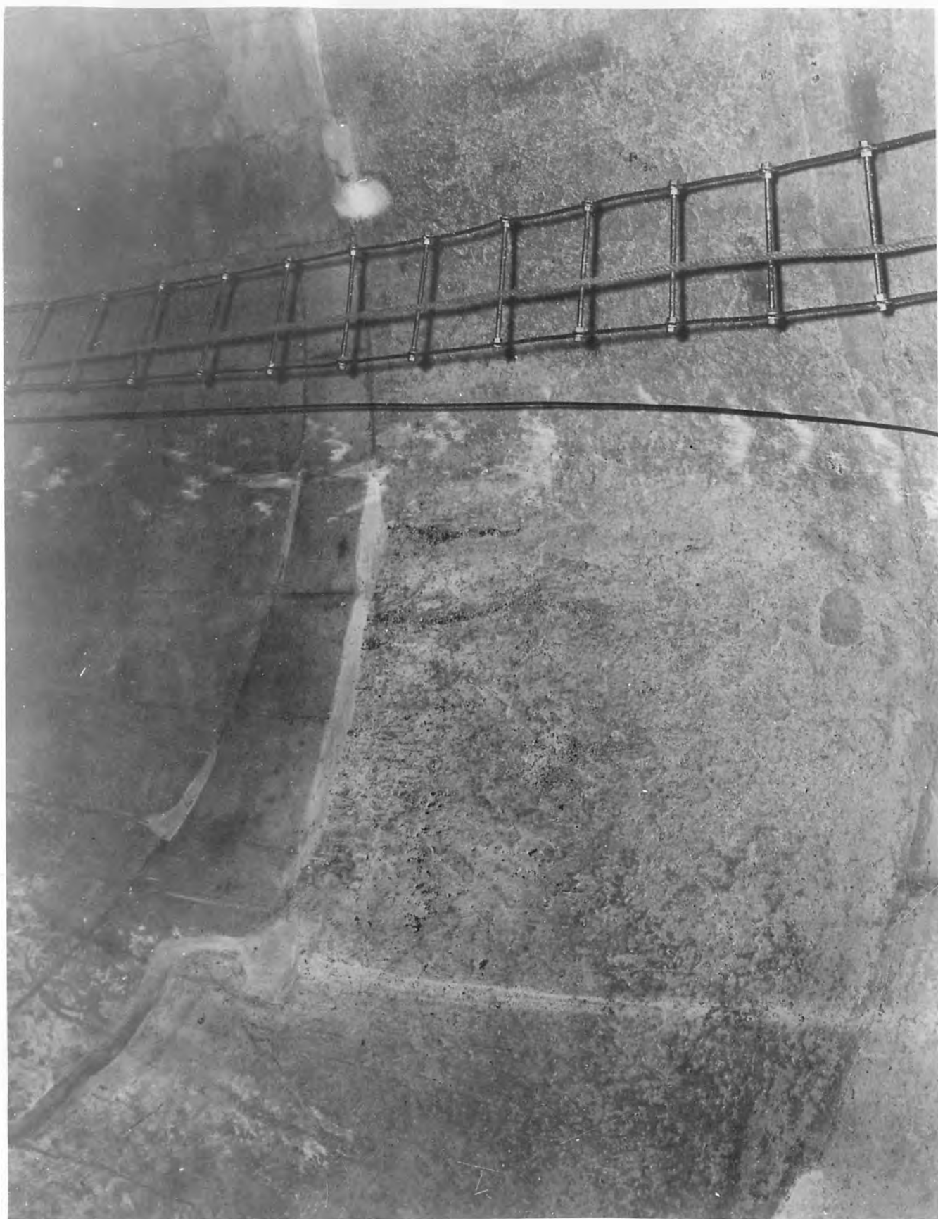
Fig. 8. Photograph 13043-3, June 7, 1945: View from draft tube floor showing pitting by cavitation at the junction of the anchor block with the old construction in the vertical curve at the right side of the R-9 draft tube entrance below the transition elbow after operation of the R-9 outlet for tests on May 25 and June 5, 1945.
