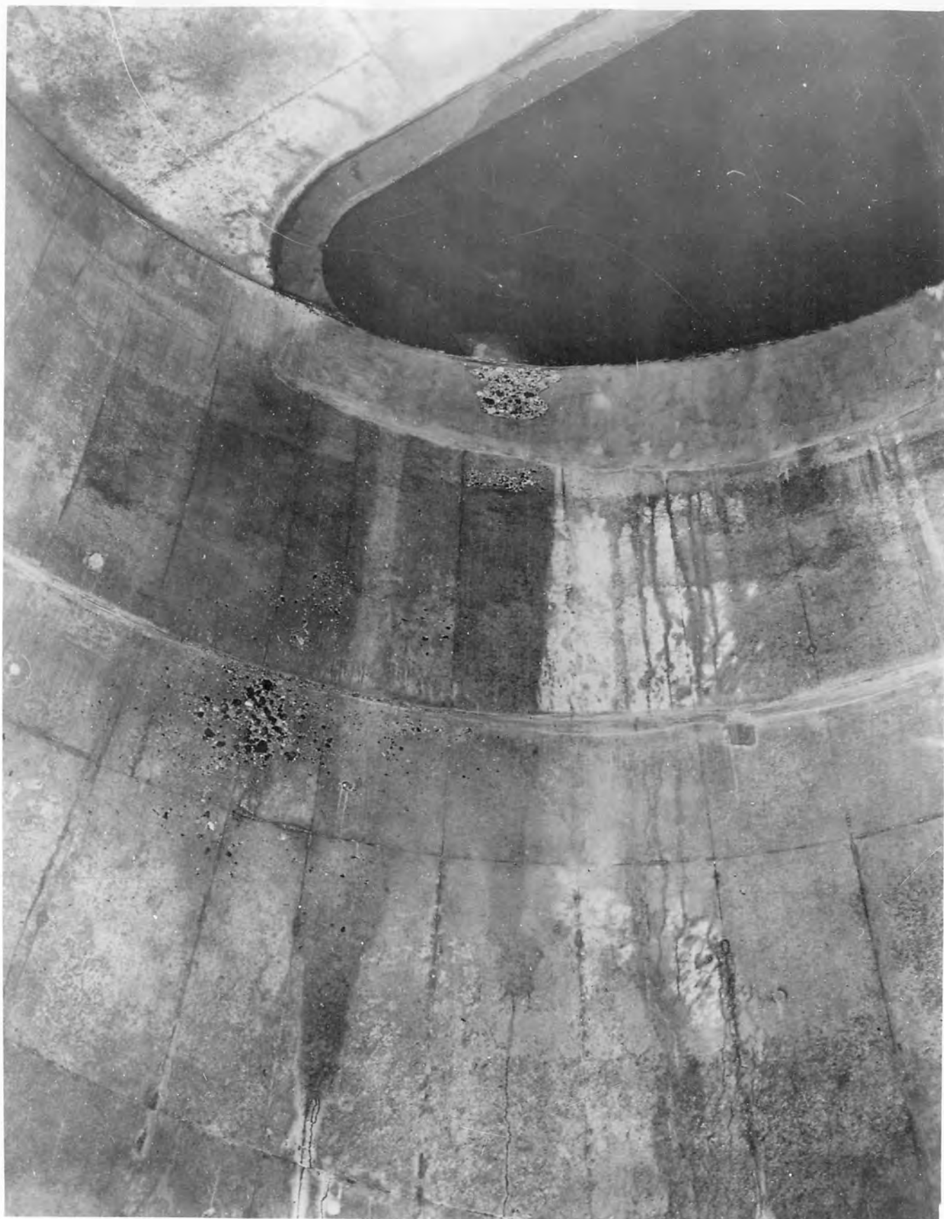
Fig. 4. Photograph 13042-3, June 7, 1945: View from draft tube floor showing pitting by cavitation in the inner curve at the right side of the steel elbow and in the wall of the anchor block below after the operation of the R-9 outlet for tests on May 25 and June 5, 1945.
