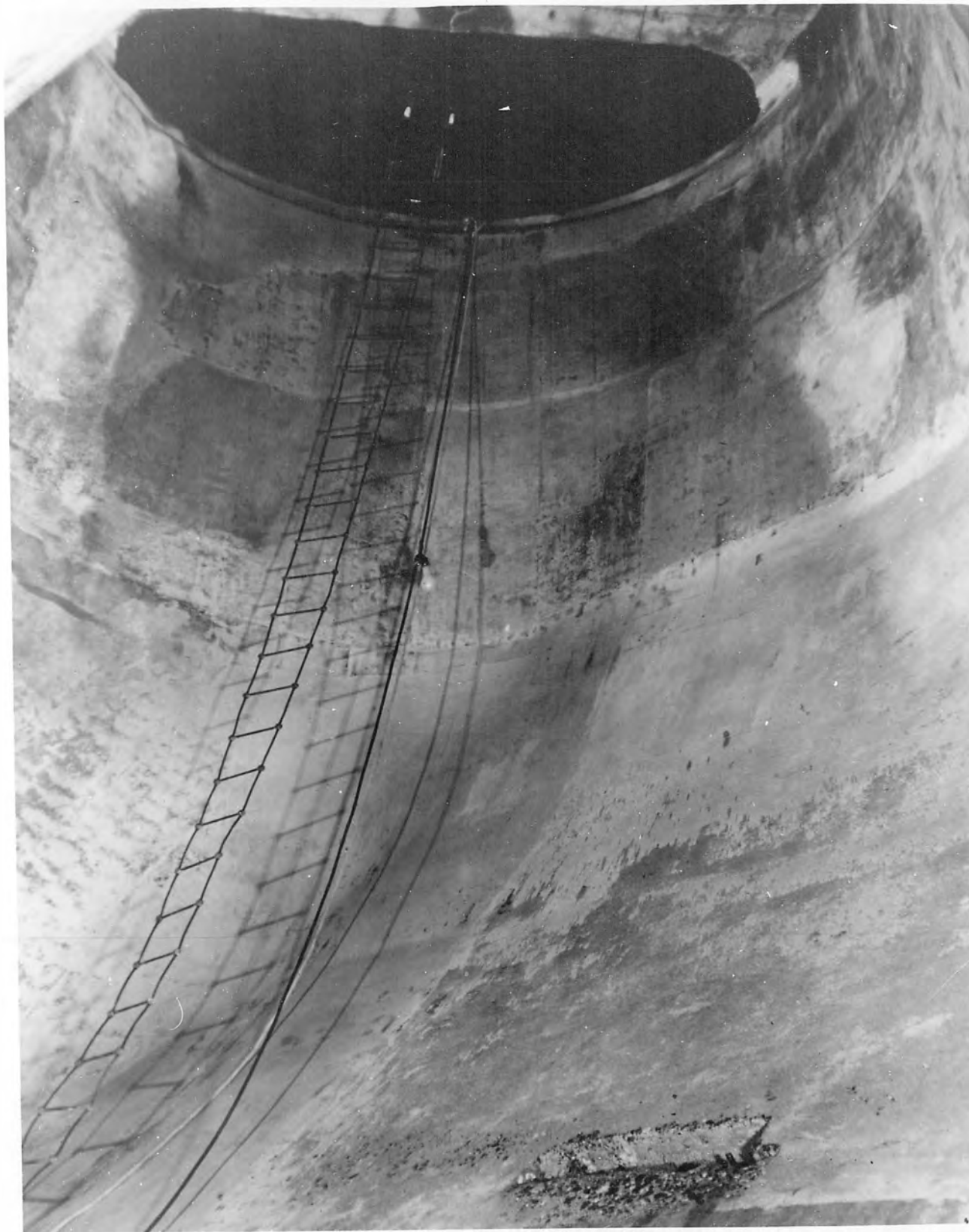
Photograph 4930-2, August 8, 1945: View from draft tube floor showing extent of cavitation in wall of anchor block at back of draft tube and near the recess from which a concrete patch had been torn during operation of the R-9 outlet for approximately 6 hours at full capacity on August 7, 1945.
