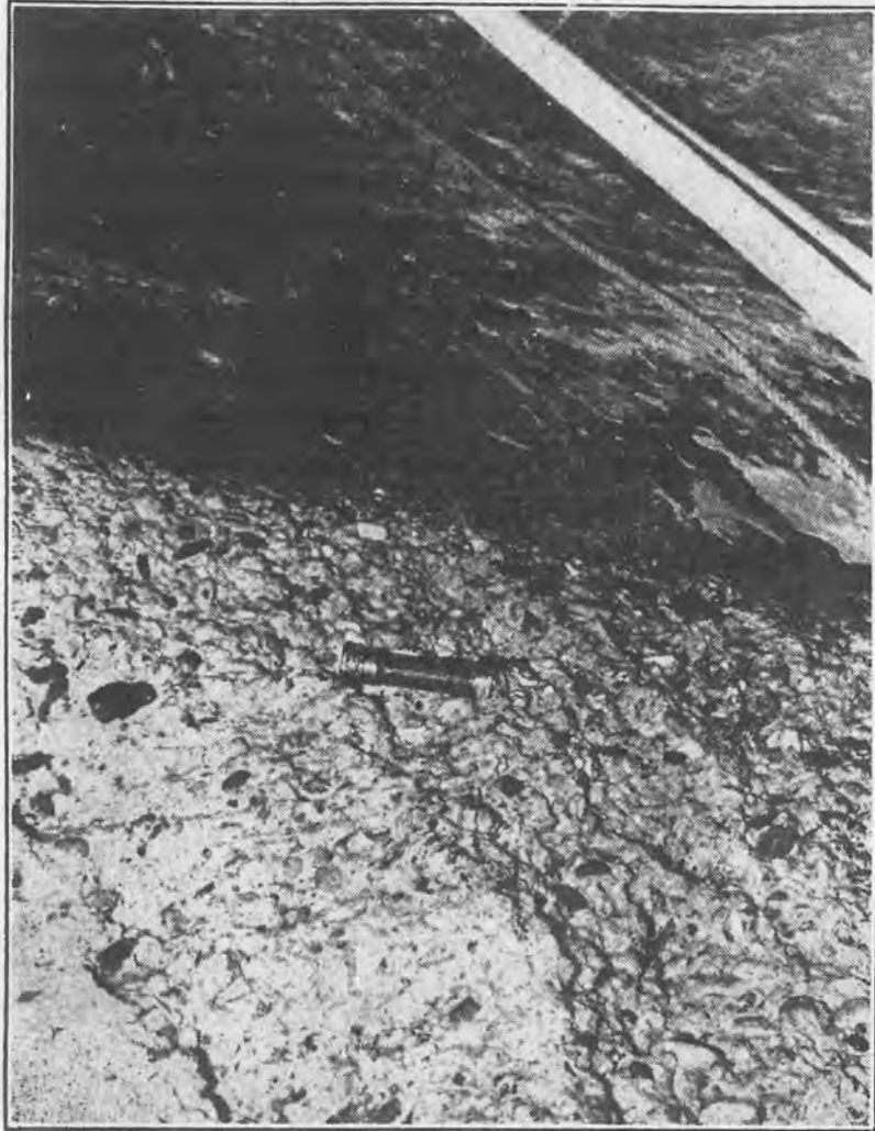
FIG. 44.—PITTED SURFACE DOWNSTREAM FROM THE MISALINEMENT IN THE TUNNEL AT THE UPSTREAM END OF THE ERODED AREA
