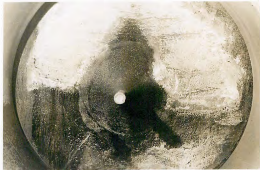
D. Extensive welding on face of needle and leakage through needle - December 17, 1941.
