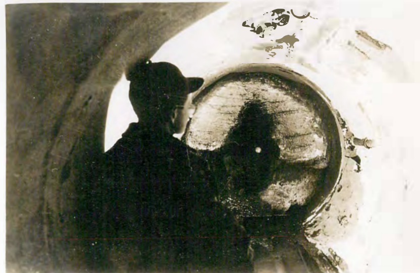
B. Extent of erosion in east valve of December 17, 1941, showing 2-inch pipes uncovered in crown and left side of conduit.
