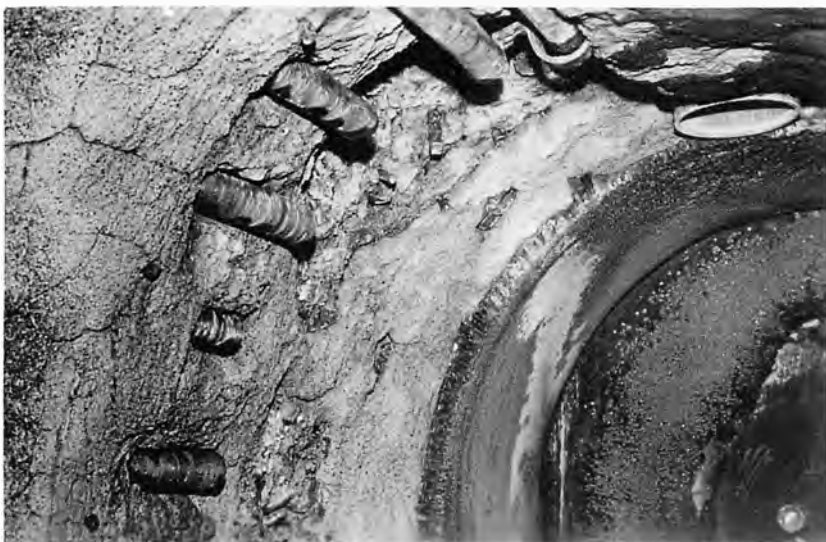
C. Remains of 2-inch air pipes and 8-inch vent and deep hole cut in right side of 52-inch conduit downstream from west 58-inch balanced valve.
