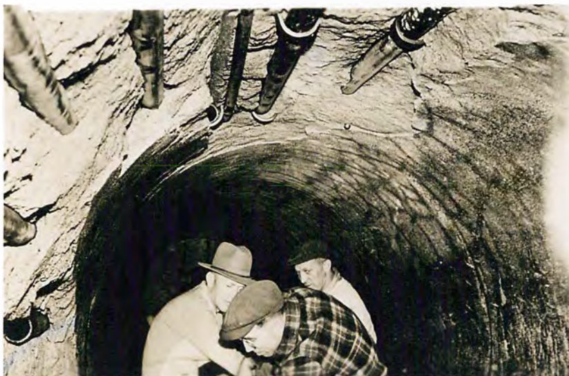
C. Two-inch air pipes laid bare by destruction of concrete downstream from east 58-inch balanced valve.
