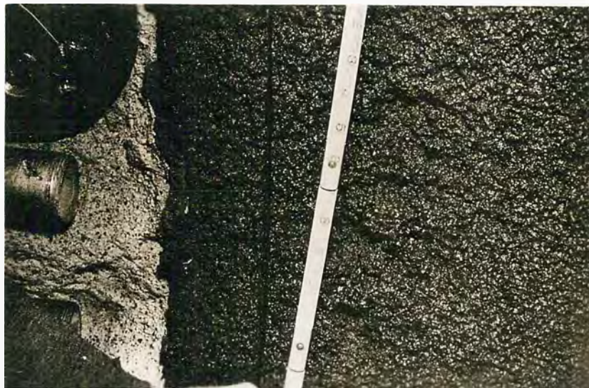
D. Severe pitting due to cavitation on conduit liner immediately below east 58-inch balanced valve.
