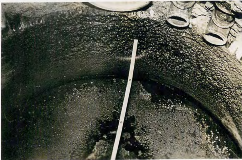
A. Severe pitting of metal liner and concrete in crown of conduit immediately downstream from west 58-inch balanced valve.
