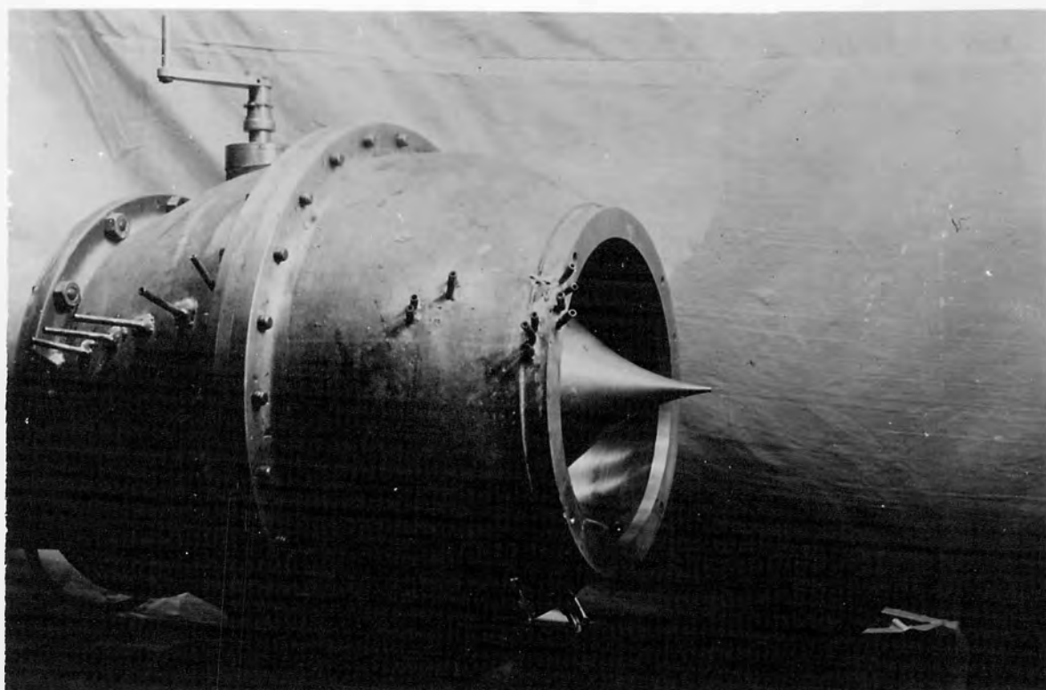
NEEDLE IN OPEN POSITION
