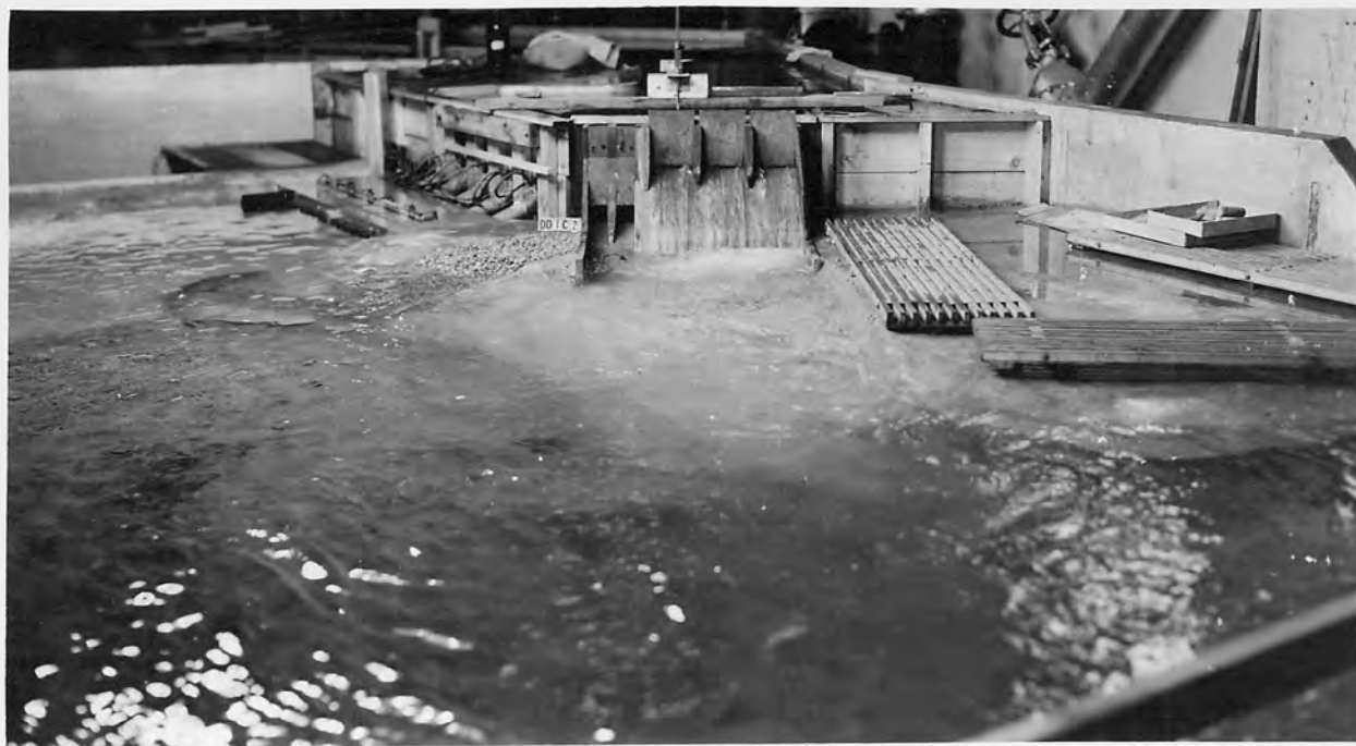
3. EDDY ON OUTLET BUCKET WHEN POWERHOUSE DISCHARGE IS 25,000 SECOND-FeET, NO OUTLET DISCHARGE, SPILLWAY DISCHARGE 25,000 SECOND-FeET.
