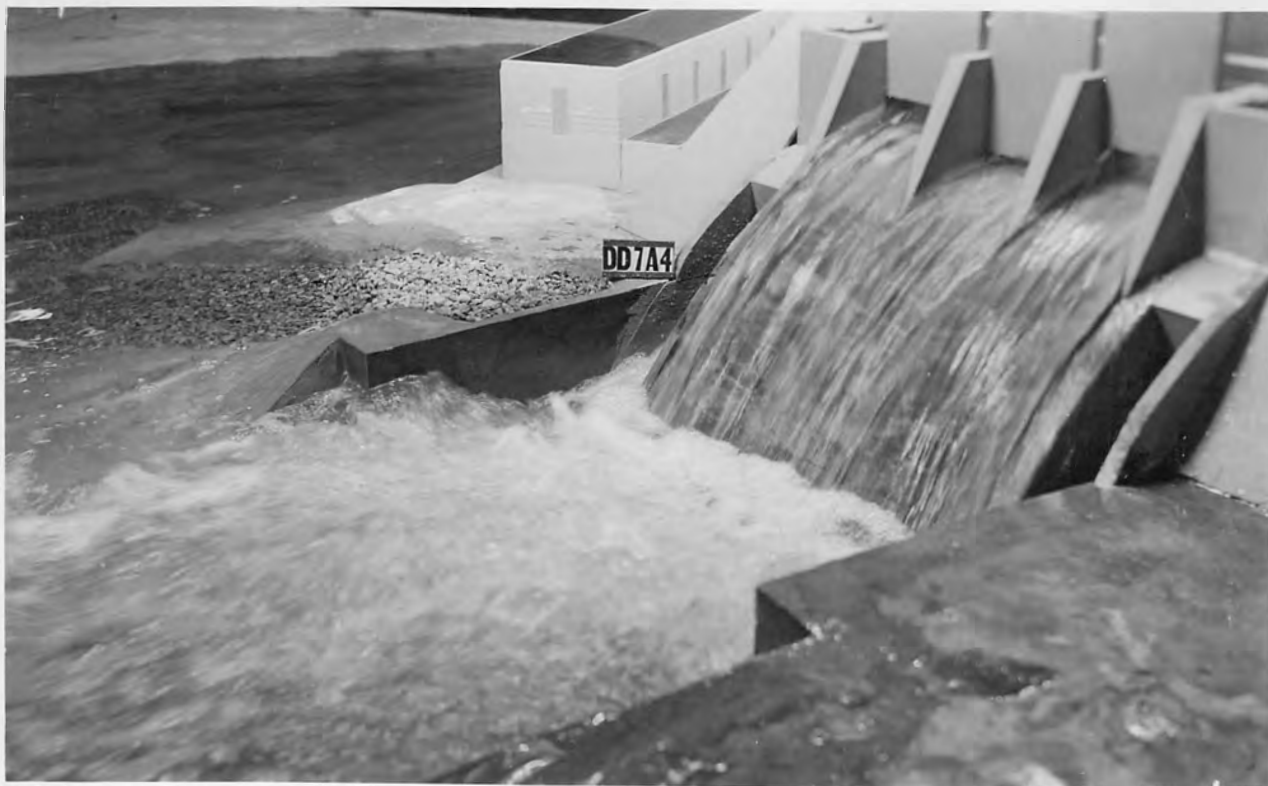
A. POWERHOUSE DISCHARGE 25,000 SECOND-FEET, SPILLWAY DISCHARGE 100,000 SECOND-FEET PRESENT TAILWATER ELEVATION, OUTLET GATES CLOSED.
