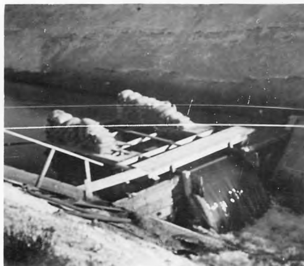
D - Eight-foot measuring weir.
