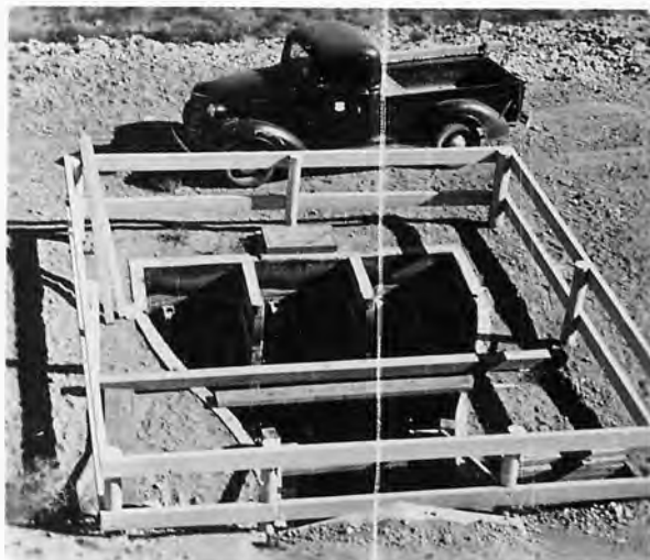
E - Open transition and 36-inch check gates.
