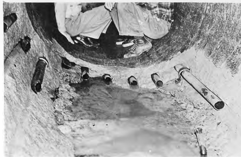
B - Remains of 2-inch air pipes in vent of 52-inch conduit looking downstream from east valve.
