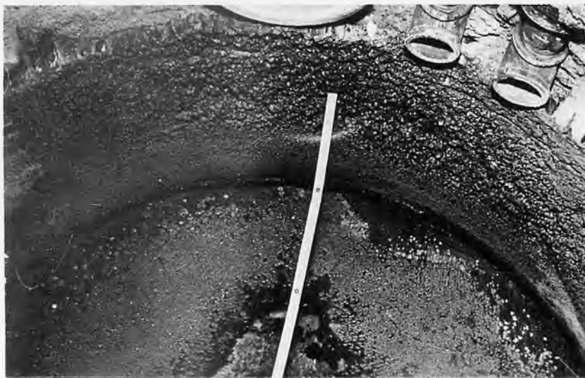
A - Severe pitting of metal liner and concrete in crown of conduit immediately downstream from west 58-inch balanced valve.
