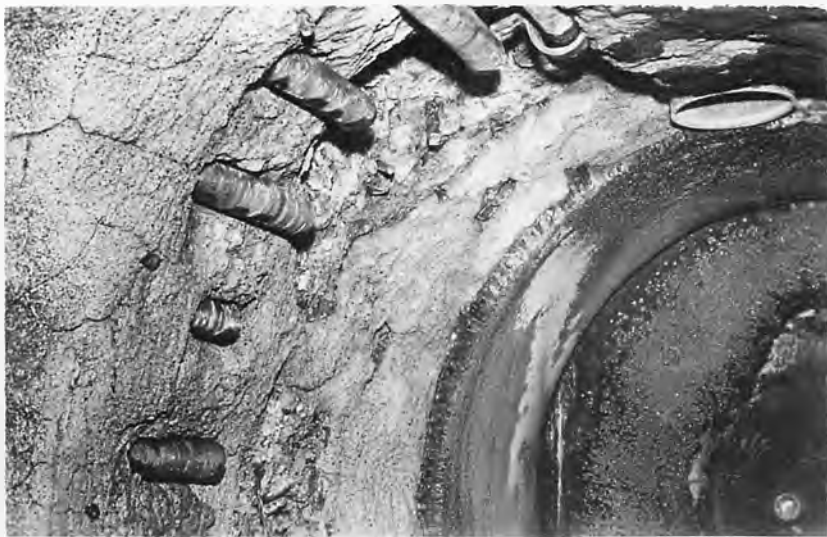
C - Remains of 2-inch air pipes and 8-inch vent and deep hole cut in right side of 52-inch conduit downstream from west 58-inch balanced valve.
