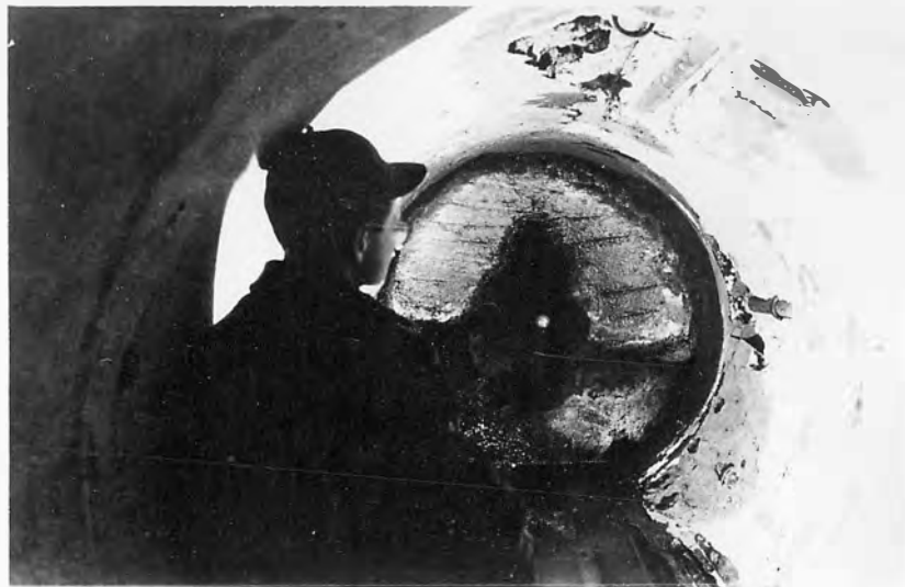
B - Extent of erosion in east valve on December 17, 1941, showing 2-inch pipes uncovered in crown and left side of conduit.
