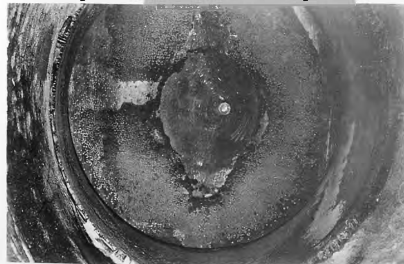
D - Face of needle in west 58-inch needle valve showing extensive welding and exposure of air vent pipes downstream from metal liner.
