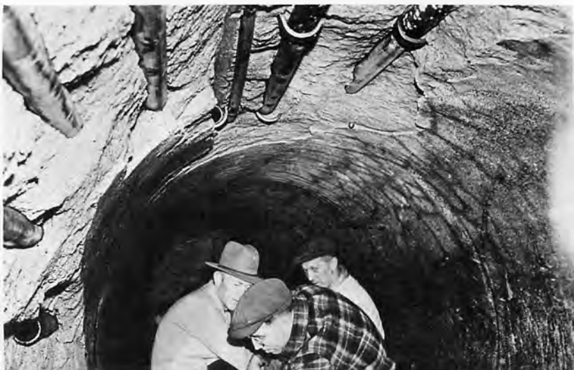
C - Two-inch air pipes laid bare by destruction of concrete downstream from east 58-inch balanced valve.
