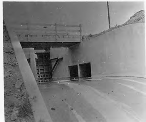
AUTOMATIC SIPHON OUTLETS BELOW WASTEWAY GATES
