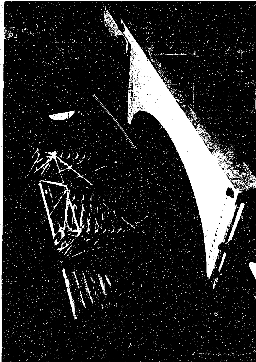
Figure 5 - Gate in position at tunnel portal.
