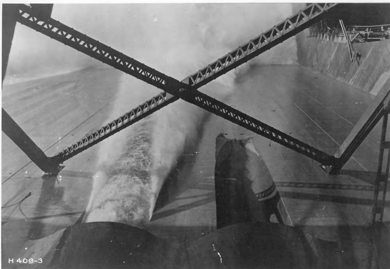
Figure 4 - Upper Outlet - Discharge 2,400 Second-Feet.
