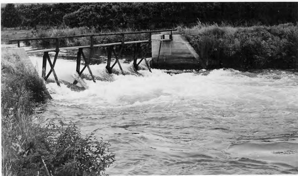
Prototype (Sunnyside Main Canal) Fig. 1. - Check Drop Before Revision - Discharge 1,300 Second-Feet
