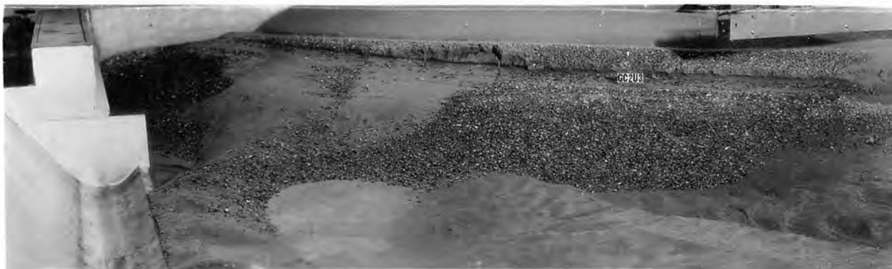
AFTER DISCHARGE OF 750,000 SECOND-FEET.
