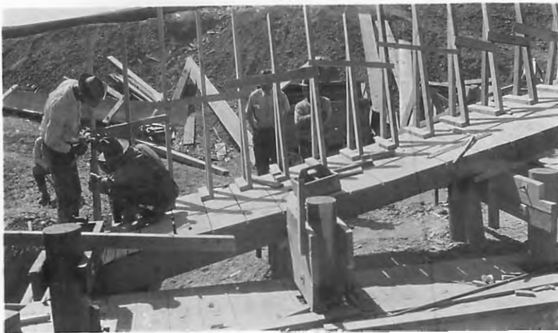
A-FLOOR SUPPORTING REAR WALL AND OGEE CREST RIBS
