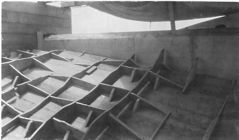
A-SLOPING FLOOR SUPPORTING TOPOGRAPHY WITH TEMPLATES
