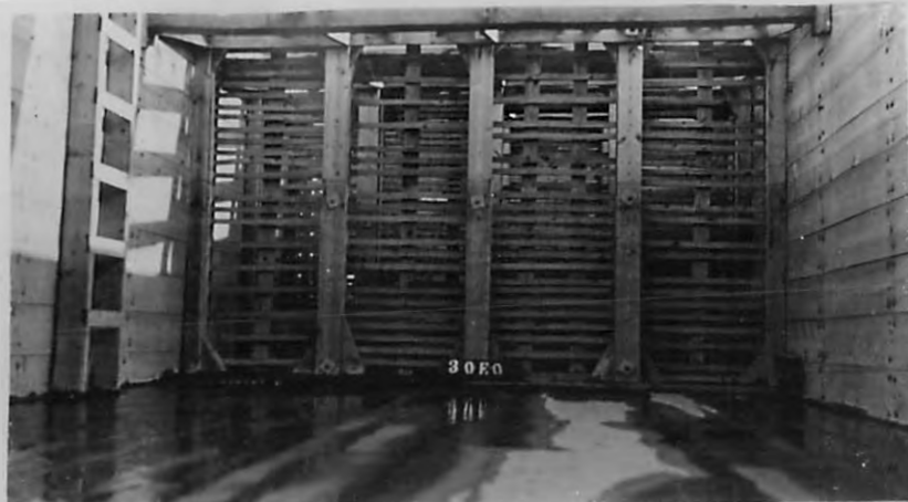
A- WEIR CHANNEL BAFFLES
