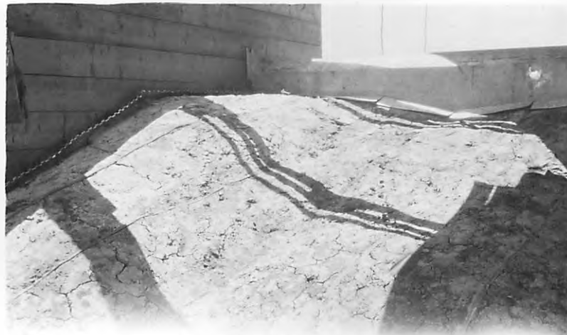
B-RAMMED CLAY FILLING AND WATER SEAL STRIPS
