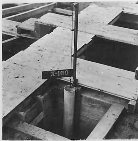
A-FLOAT GAGE FOR INDICATING HEAD ON WEIR
