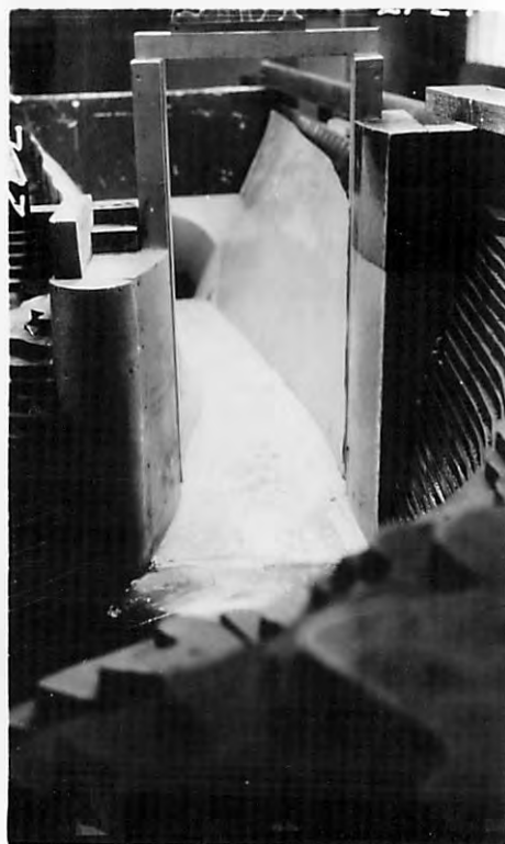
C- ROUNDED NOSE ON GATE PIER
