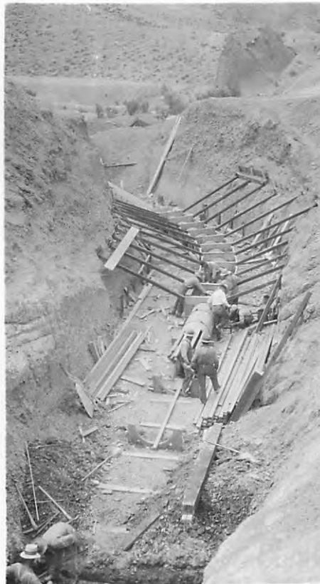
B-CONSTRUCTION OF HORIZONTAL BEND
