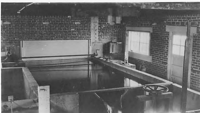
C THE WEIR BOX AND MEASURING WEIR
