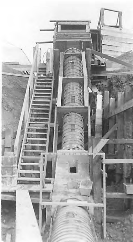
A-INCLINED TUNNEL & VERTICAL BEND
