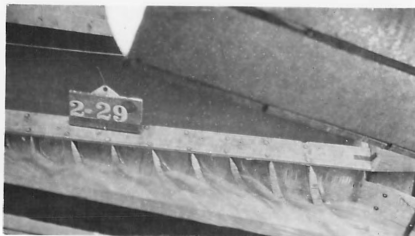
D-DISCHARGING SIDE CHANNEL WITH VANES ON THE CREST
