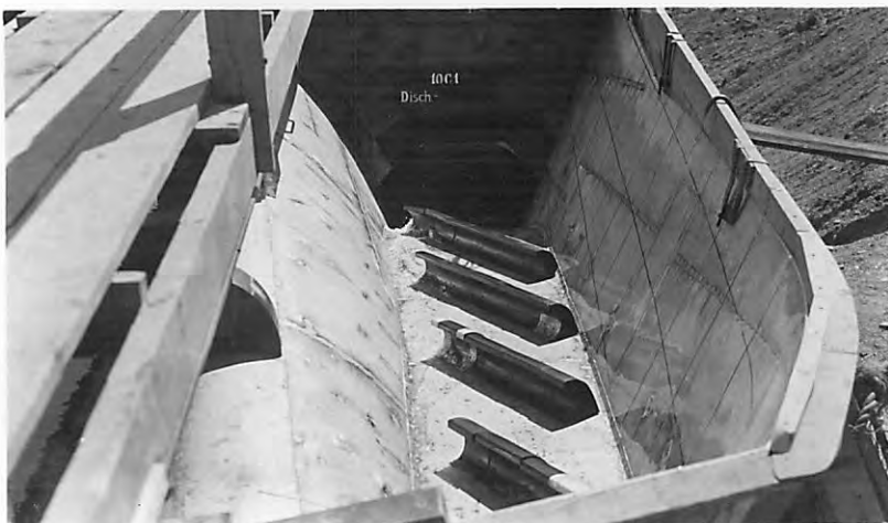
C-NO DISCHARGE - BAFFLES INCLINED UPSTREAM
