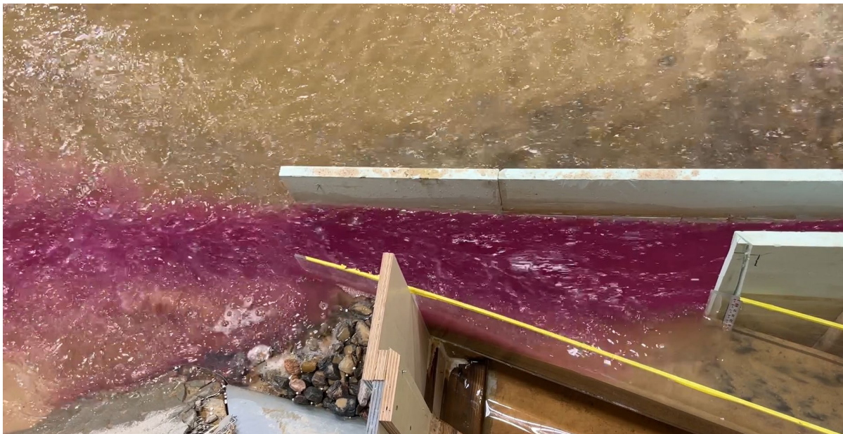
Figure 20. Downstream end of flushing channel open at river flow of 6,000 ft 3 /s. The desander sluice is closed and there is little recirculation in the vicinity of the desander exit.
