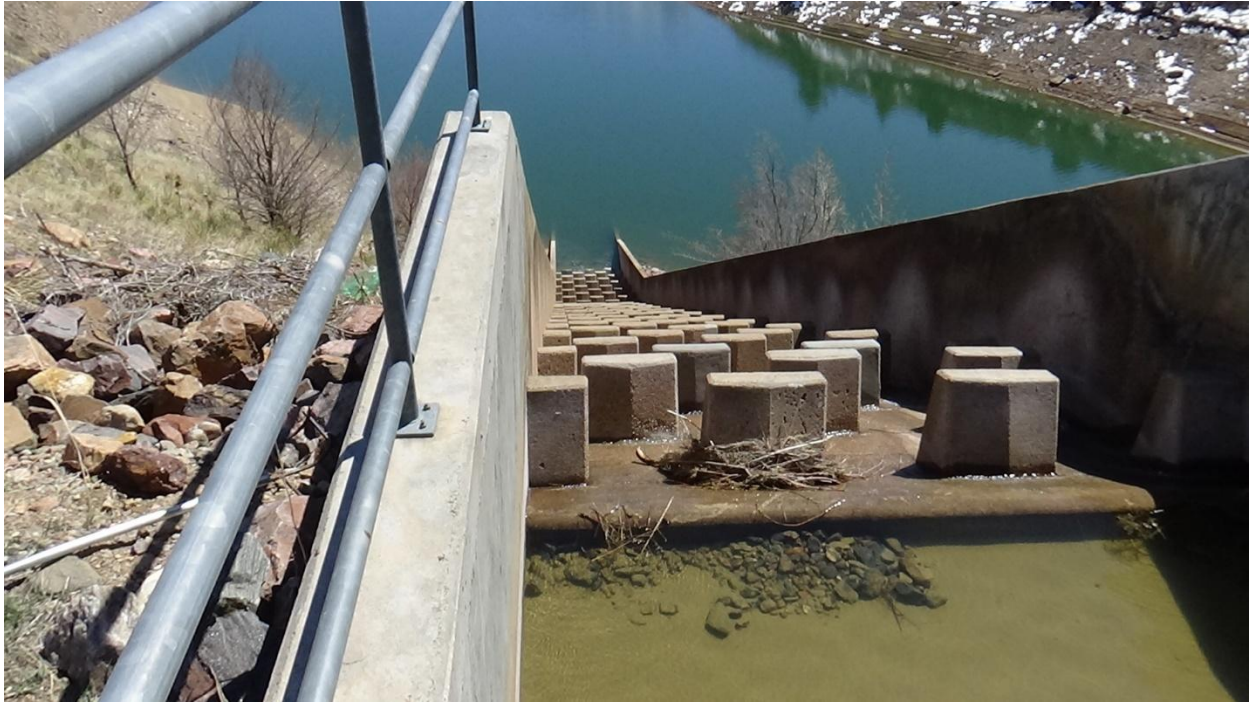
Figure 25 Downstream of Zone A flume, looking down the “dragon tooth” spillway that discharges into Ralston Reservoir.
