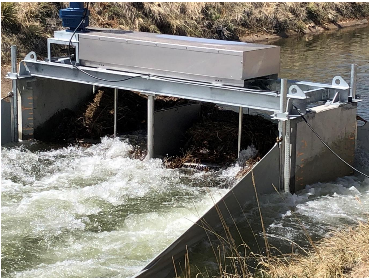
Figure 20 Debris clogged in the HK rotors. Looking upstream.
