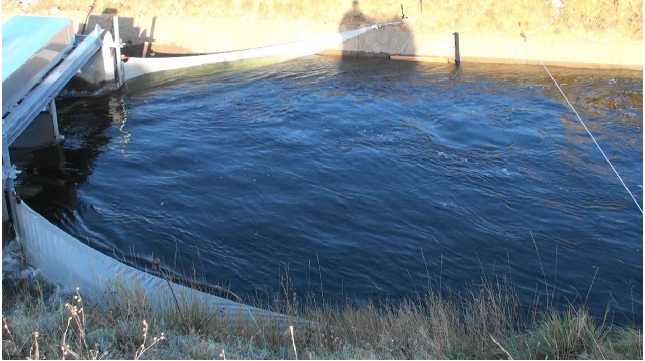
Figure 12 Water level upstream of HK #5 (station 250) at 266 ft 3 /s. Flow is from right to left.
