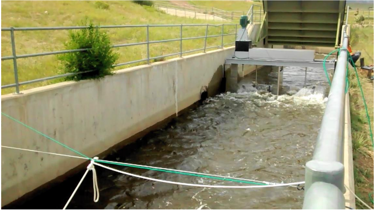
Figure 30 HK #3 operating near the upstream end of Zone A, looking upstream. A radial gate is located just upstream from HK #3.
