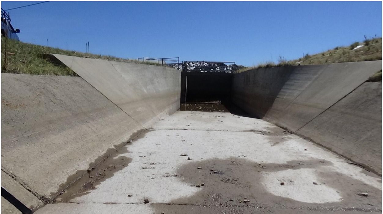
Figure 32 Trapezoidal to rectangular transition at the downstream end of Zone B, looking downstream.
