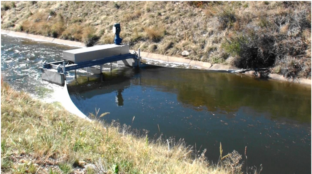
Figure 13 Water level near top of lining upstream of HK #9 (station 890) at 266 ft 3 /s. Flow is from right to left.
