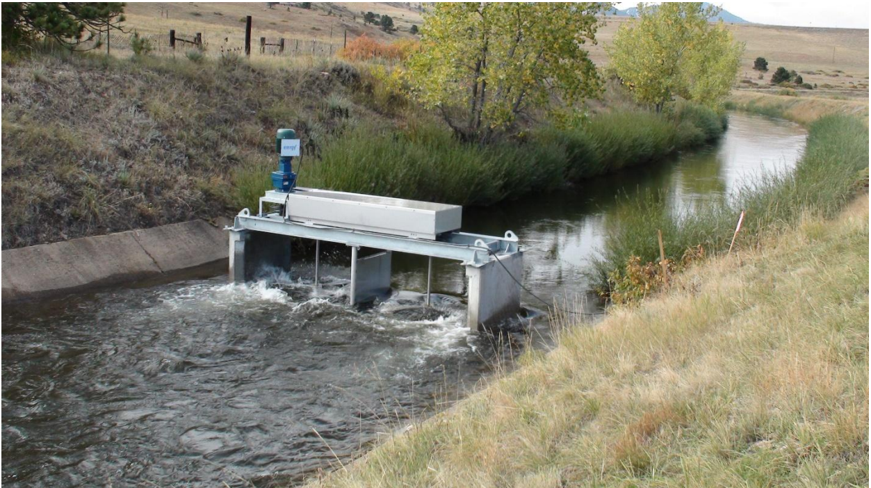
Figure 38 HK #10 with no transitions (Zone B station 2,045 ft at connection with Zone C) operating at 266 ft 3 /s, looking upstream.
