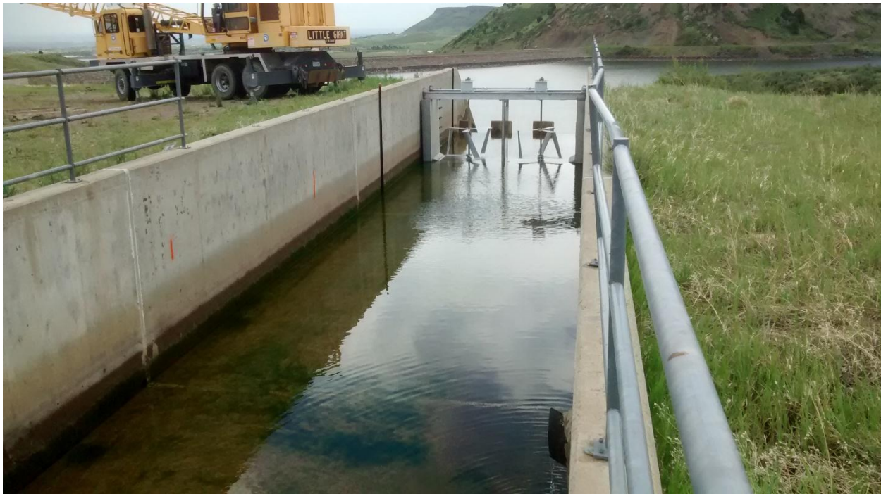
Figure 28 First HK unit installed near the downstream end of Zone A, looking downstream.
