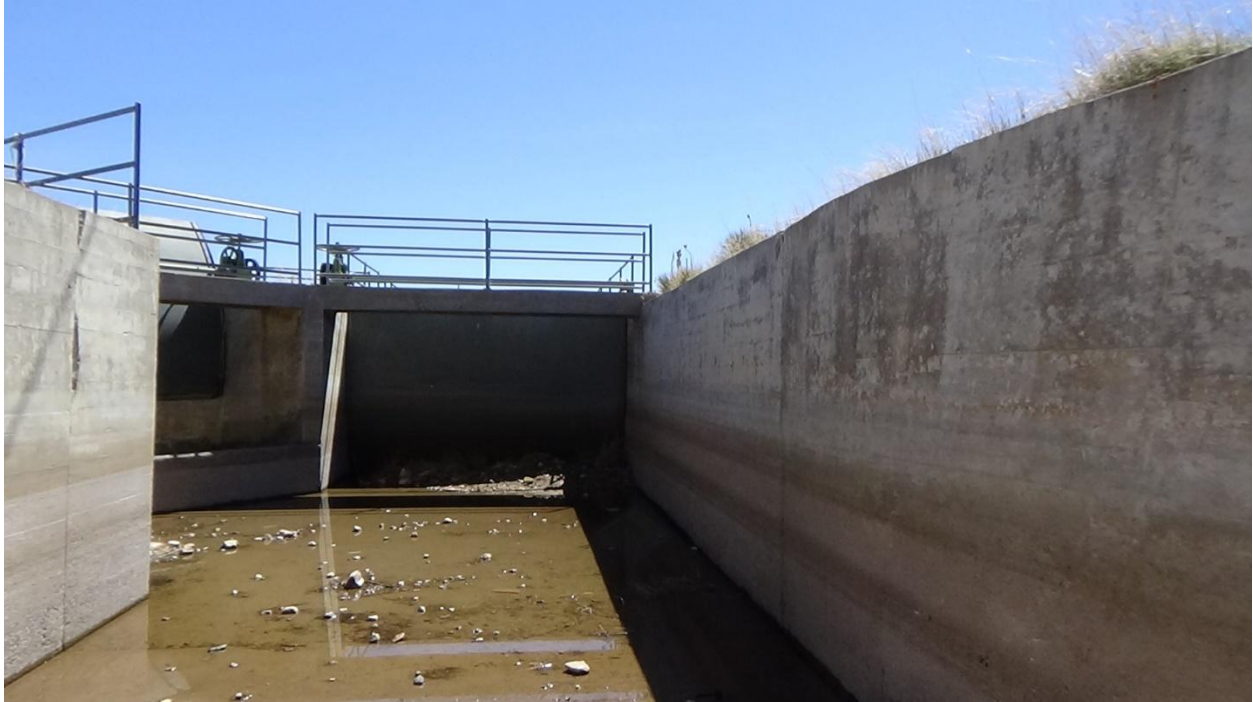
Figure 31 Bifurcation structure at downstream end of Zone B. The left leg goes to the Zone A flume and the right leg (straight) leads directly to Ralston Reservoir.
