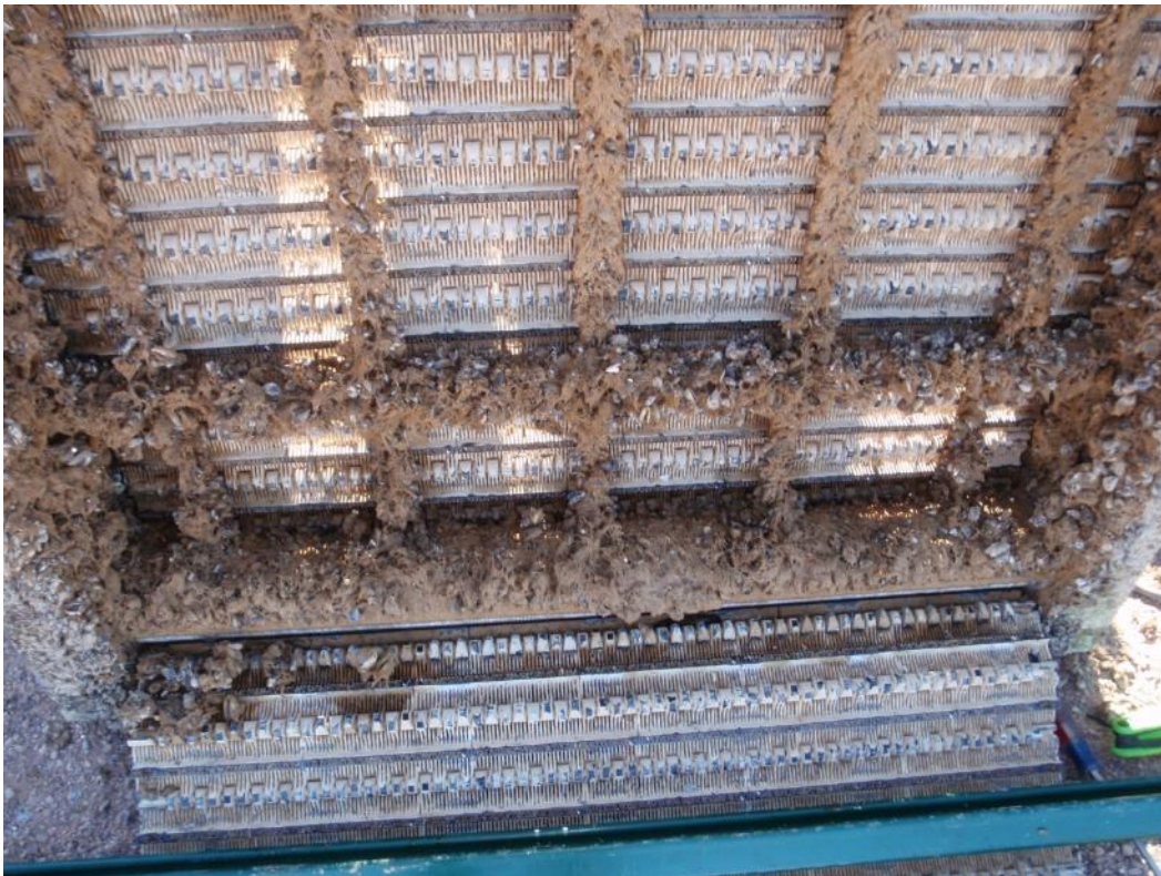
Figure 17 Inside of the Hydrolox traveling screen after 2 years of operation at Lake Mead.
