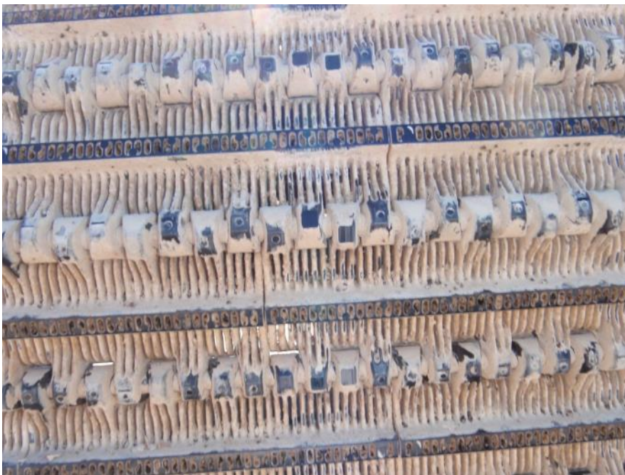
Figure 37 Biofilm built up on the Hydrolox screen (inside of screen looking out).
