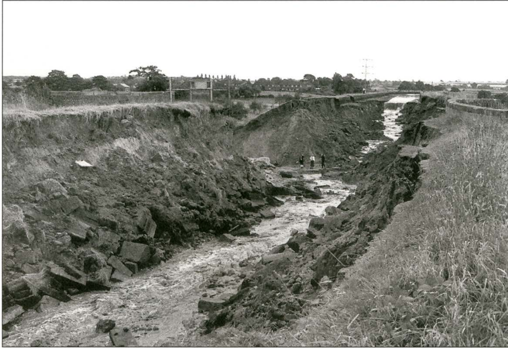
Figure 9. — Breach of the River Bollin embankment and aqueduct in 1971, United Kingdom. Note headcut in the distance, migrating up the canal (upper right). A similar headcut is located behind the photographer's position. Photo courtesy of Mark Morris, HR Wallingford.
