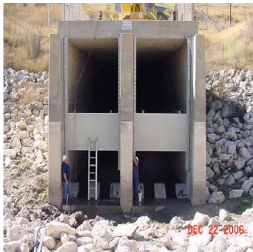
Figure 33. — Installation of Choke Canyon stilling basin deflectors in December 2006.
