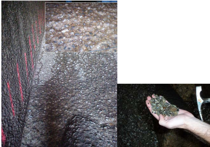
Figure 2. — Typical abrasion damage (Choke Canyon stilling basin).
