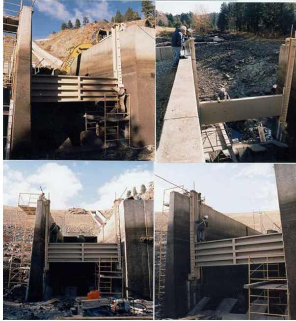
Figure 32. — Installation of first prototype deflector at Mason Dam in Oct 2002
