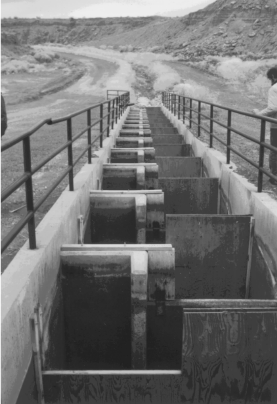
Figure 4 – Current intermediate fish ladder baffles with FWS modifications
