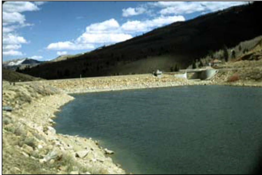
Figure 14. —Scofield Dam, Utah.
