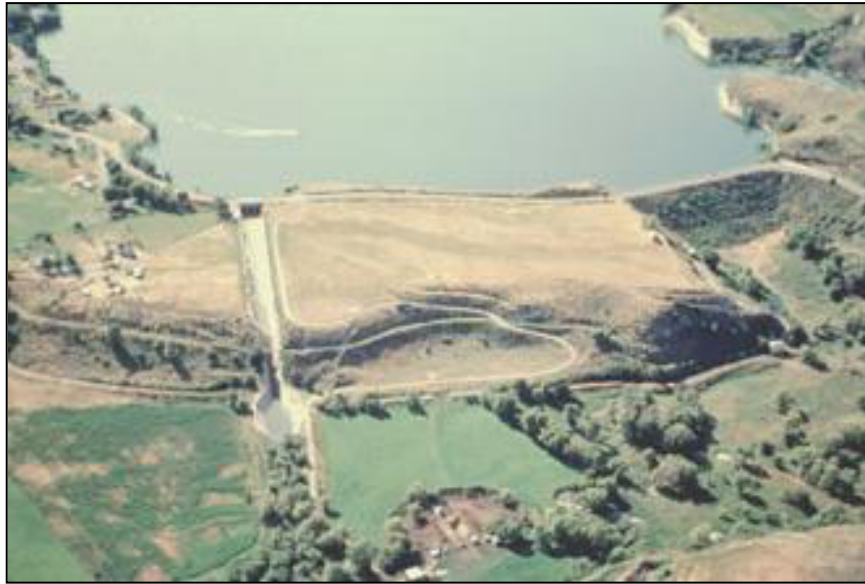
Figure 15. —Hyrum Dam, Utah.
