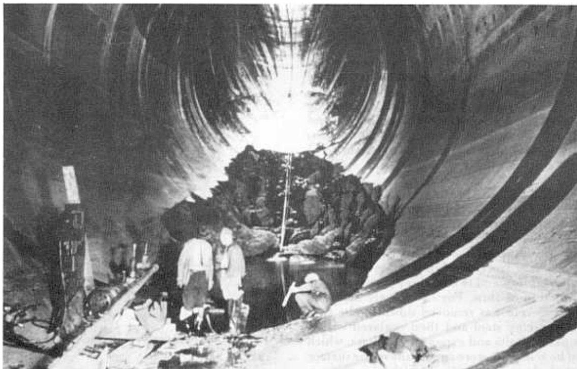
FIGURE 7-7.—Hoover Dam, Arizona tunnel spillway — major damage (1942).
