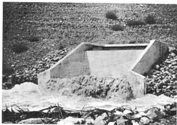
Picacho North Dam outlet works structure discharging 210 c.f.s. (80 percent of maximum capacity).
