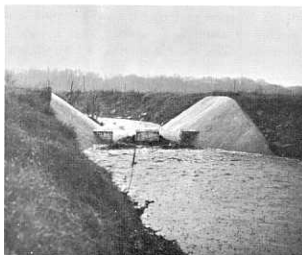
Performance of structure during rainstorm. Discharge 81 c.f.s. in May 1959. Design discharge 400 c.f.s.
