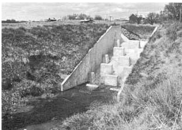
Structure after 4 years of operation. Performance has been satisfactory. Design discharge 625 c.f.s.
