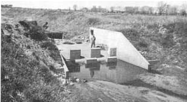
No flow through structure on Bostwick Courtland Canal, Drain A, Sta. 6+08, designed for 924 c.f.s.
