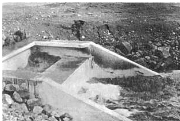
South Dam outlet works structure discharging 130 c.f.s. (80 percent of maximum).
