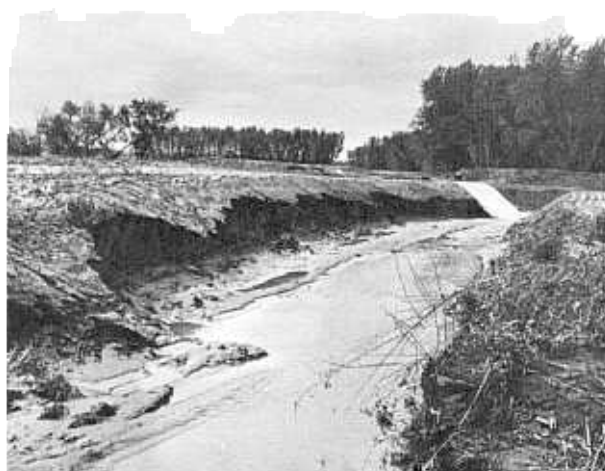
Upstream banks were badly eroded.
