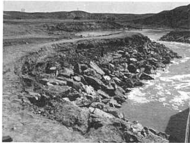
FIGURE 174.—Surge-type waves extracted fine earth material from behind coarse riprap, causing entire mass to settle away from top of bank. High water line was below elevation where man stands.
