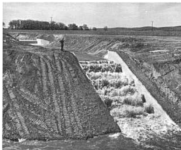
Baffled apron of Culbertson Canal Wasteway 3.3 discharging 75 c.f.s. Good performance. Design discharge 400 c.f.s.
