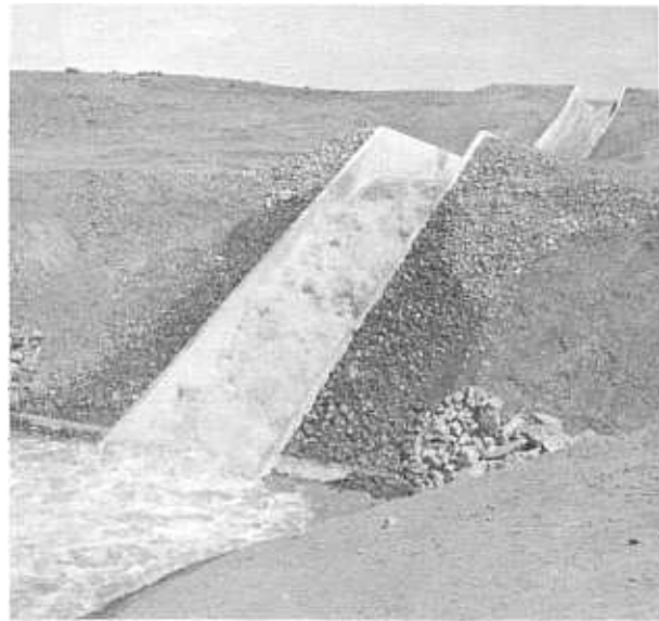
Dark rock area adjacent to training walls is wet from spray.
