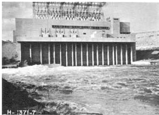
90-inch outlet works valves 100 percent open, discharging 4,500 c.f.s., approx. T.W. elevation 183.6. Turbine gates 72 percent open, 100 percent load.
