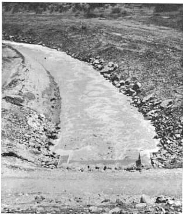
FIGURE 172.—Flow conditions downstream from Picacho South Dam outlet works are entirely satisfactory. There was no disturbance or loss of riprap under a discharge of 130 c.f.s.
