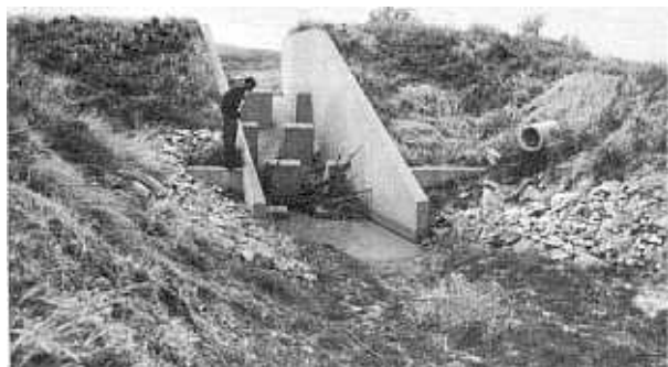
No flow in structure on Bostwick Courtland Canal, Drain A, Sta. 67+93. Trash has accumulated at foot of chute. Design discharge 277 c.f.s.
