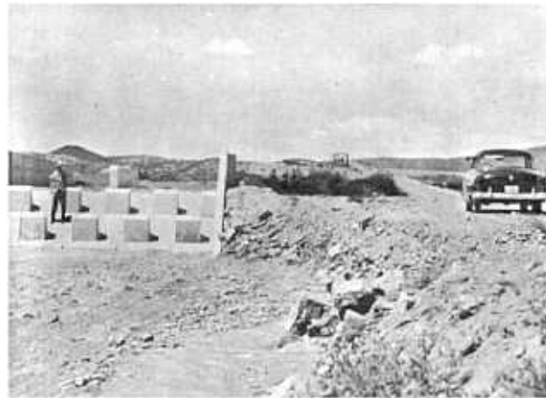
Channel after flood—material was deposited rather than scoured.
