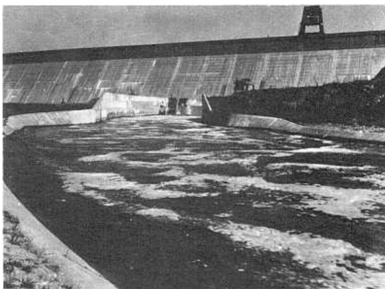
FIGURE 26.—Hydraulic performance of wave suppressor for Friant-Kern Canal.
