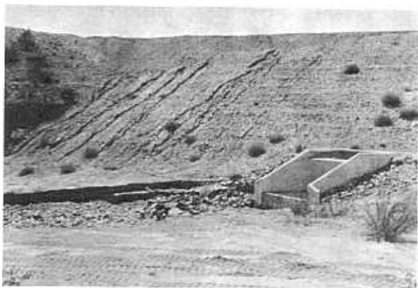
FIGURE 168.—Impact-type stilling basin structure, Picacho North Dam, following flood of August 20, 1954.
