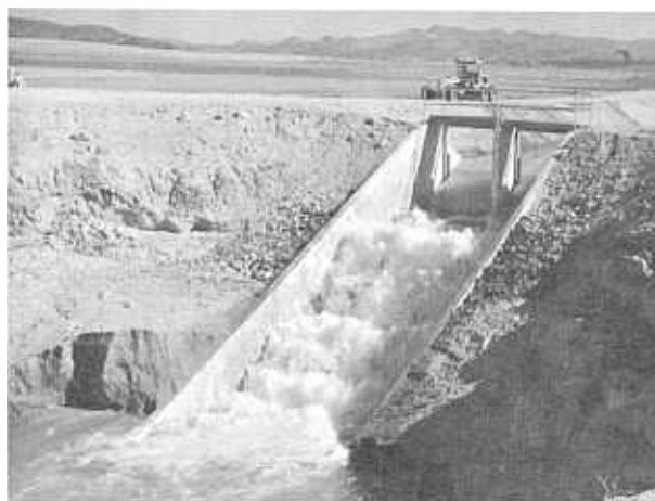
FIGURE 126.—Construction and performance of baffled chutes.
