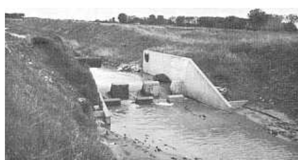
With a discharge of about 5 c.f.s., the structure performs well. It is reported that larger flows are handled satisfactorily.
