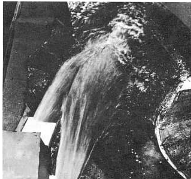
FIGURE 161 Model-prototype comparison, Fontana Dam spillway flip buckets.
