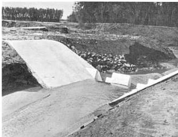
Unstable banks collapsed after only 6 months of operation. Protection was afforded by downstream riprap.
