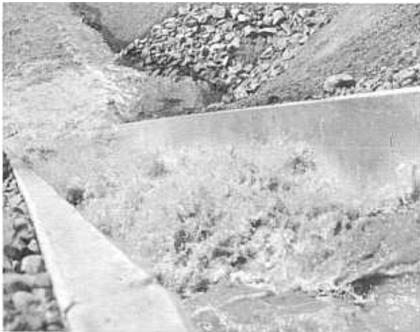
FIGURE 127.— Prototype installation of baffled chute.
