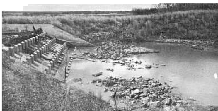
FIGURE 131.—Progress of erosion in Bostwick Crow Creek Drain, Sta. 28+90. Design discharge 2,000 c.f.s.
