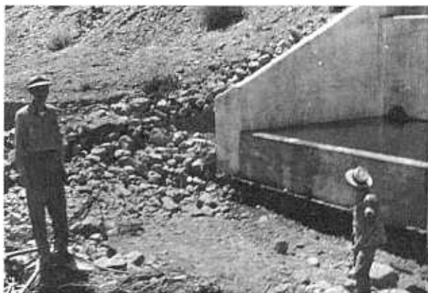
Scour below Picacho North Dam outlet works following flood of August 20, 1954. Evidence points to under-sized riprap.
