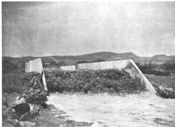
Estimated discharge 15 c.f.s. per foot width (half capacity).
