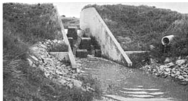
Discharge about 3 c.f.s. Reports received indicate that structure performs well for large discharges.
