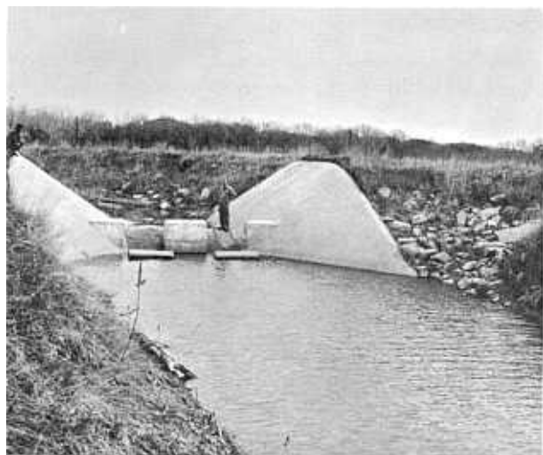
Stabilized banks in April 1959 show no evidence of erosion.
