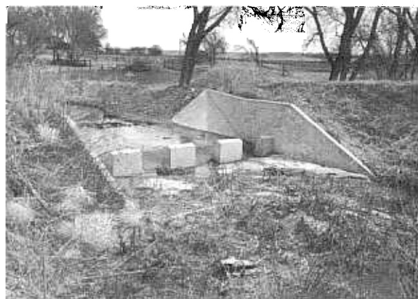
Structure after 5 years of operation. Performance has been satisfactory. Design discharge 1,100 c.f.s.
