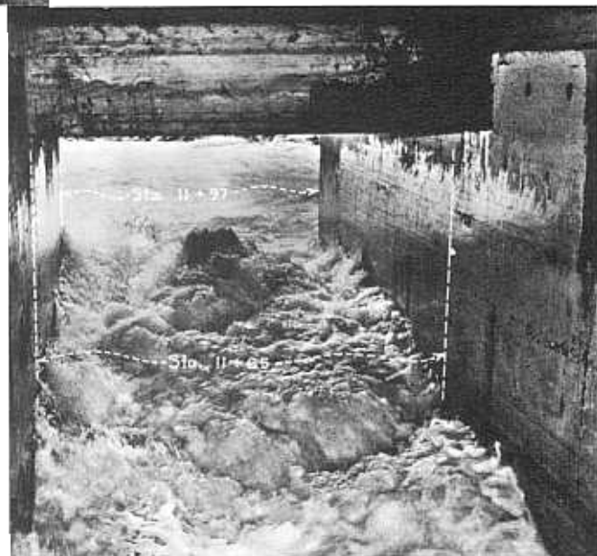
FIGURE 91.—Boysen Dam: left valve of outlet works basin discharging 732 c.f.s.—looking upstream.
