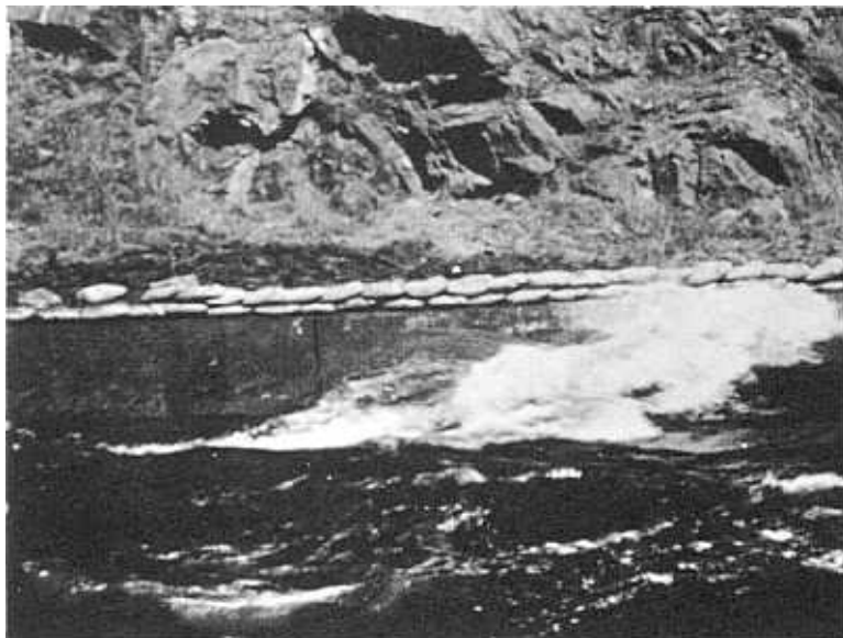
Q=3,900 c.f.s.—before wave suppressor was installed.
