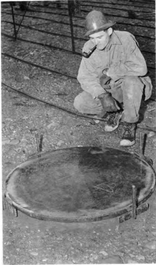
FIGURE 9 - Steel cover plate placed over pair of embedded strain meters.
