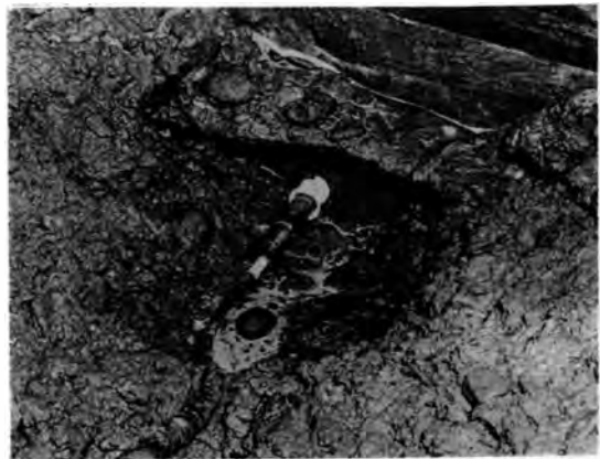
FIGURE 10 - Typical joint meter installation.
