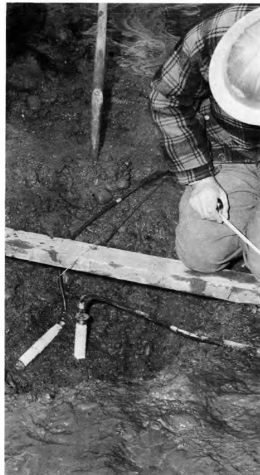
FIGURE 8 - Pair of strain meters for determining volume change in mass concrete.
