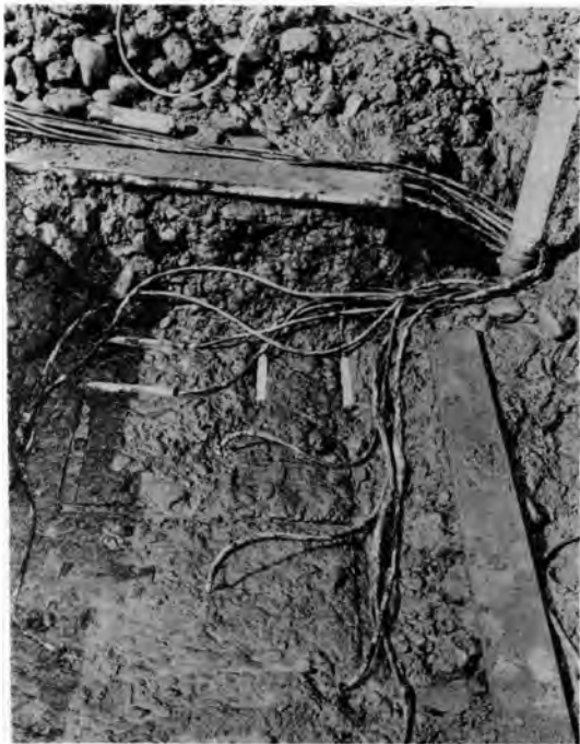
FIGURE 5 - Strain meter group at base of maximum section.
