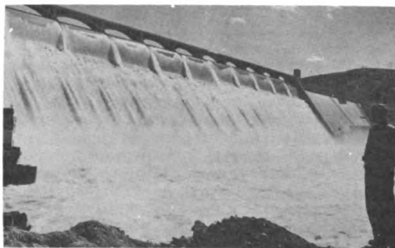
A. Spillway flow at Grand Coulee Dam passing over outlet deflectors
