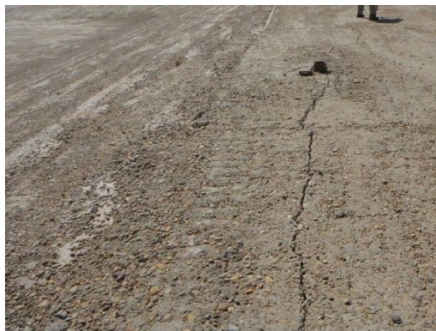
14. Longitudinal crack in dam crest near STA 8+50 and B-103, looking right from STA 8+60. This crack is about 0.25 to 0.5 inches wide and 25 feet long.
