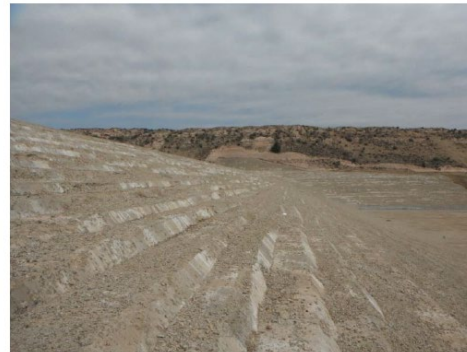
15. Downstream slope, looking left from near STA 7+50.
